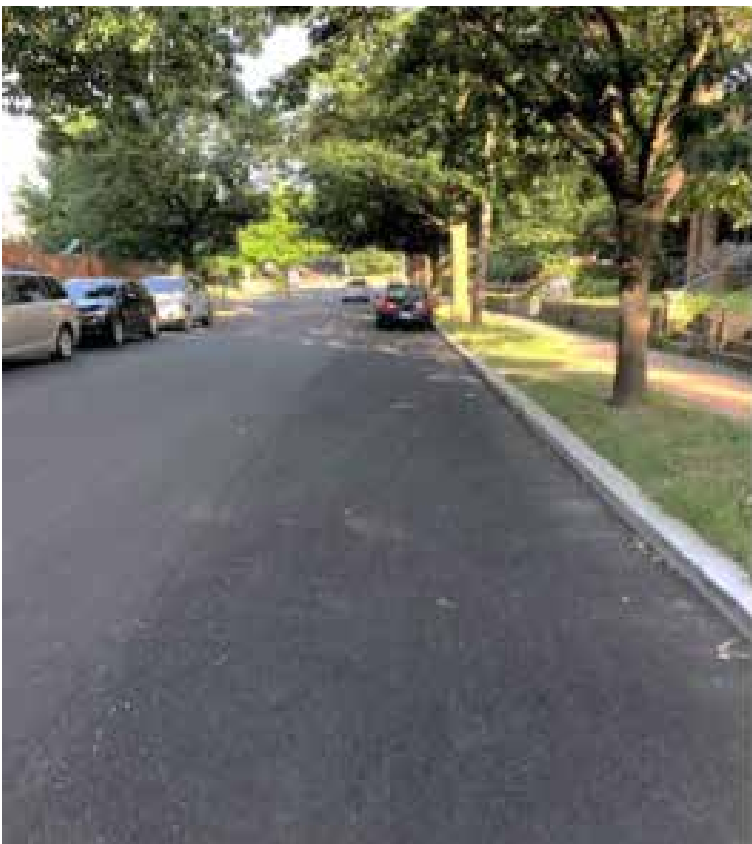
Parking lane permeable pavement. Photos and pictures courtesy of DC Water.
