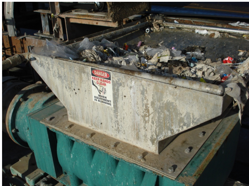
Here is a grinder pump that is installed after the bar screens. This debris is sent to the landfill.
