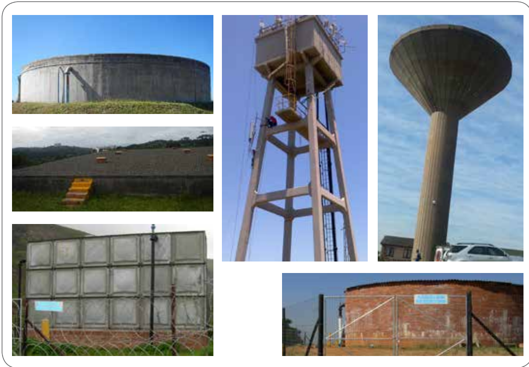
Figure 21 Examples of reservoirs and water towers
