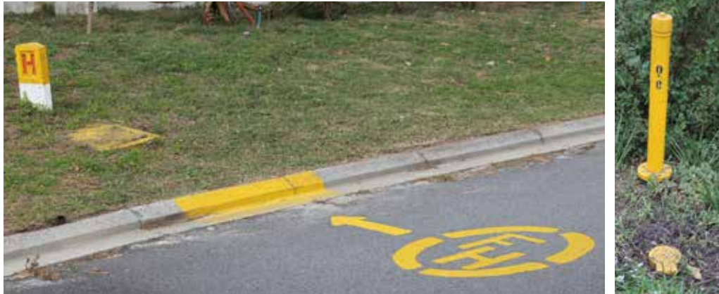
Figure 16 Examples of fire hydrants
