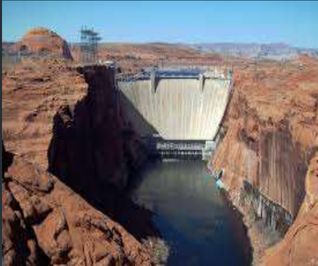
Storms water and Dams
