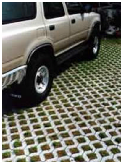
One type of alternative paver consists of a concrete lattice structure for support with grass growing in the void spaces (Source: Lo Gioco Landscaping, Inc., no date)
