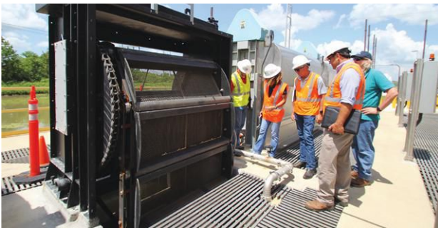
IMAGE 5: Three existing 5-foot-wide traveling screens that were well maintained were also reused.
