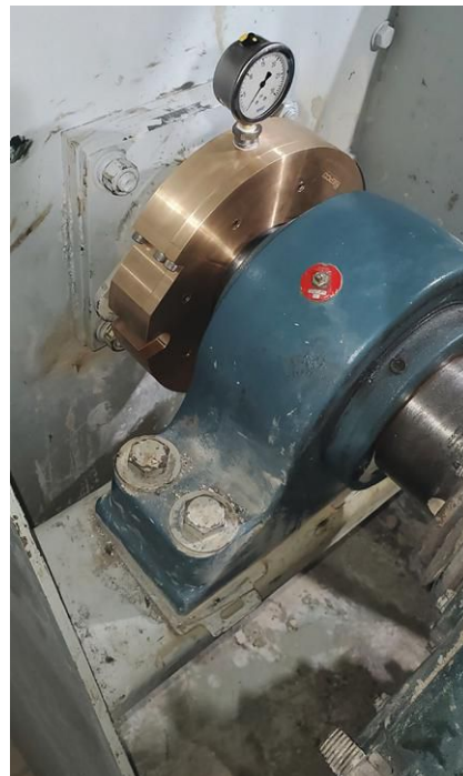
IMAGE 4: An air seal installed on the gypsum screw conveyor, which eliminated all leakage
