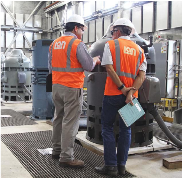
IMAGE 4: Relocating the pumps required a specific construction sequence, detailed scheduling and extensive coordination.
