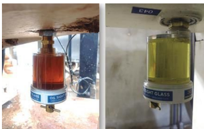
IMAGE 5: BS&W bowl showing clear oil discoloration
