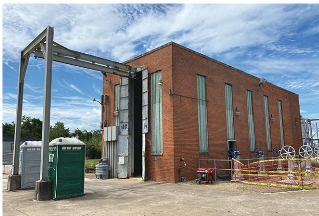
IMAGE 1: Most of the existing pump station's infrastructure needed repair or replacement. (Images courtesy of Lockwood, Andrews & Newnam)
