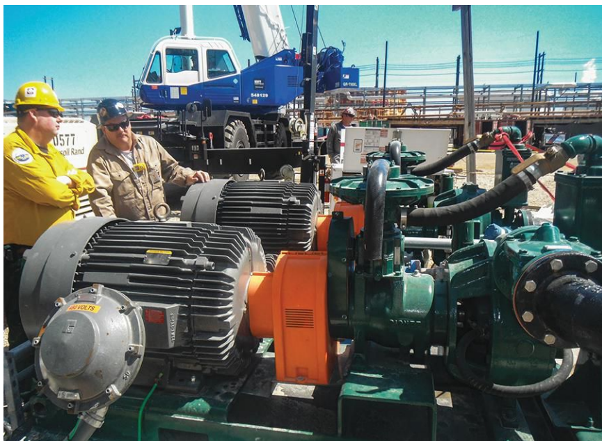
IMAGE 3: Skid system at Port Arthur, Texas, refinery site
