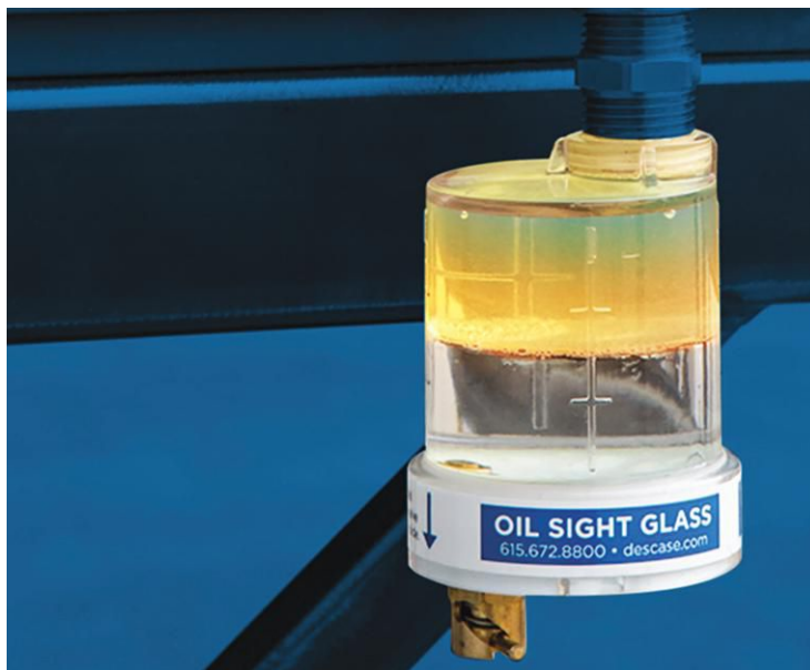
IMAGE 3: BS&W bowl showing free water inside the pump housing
