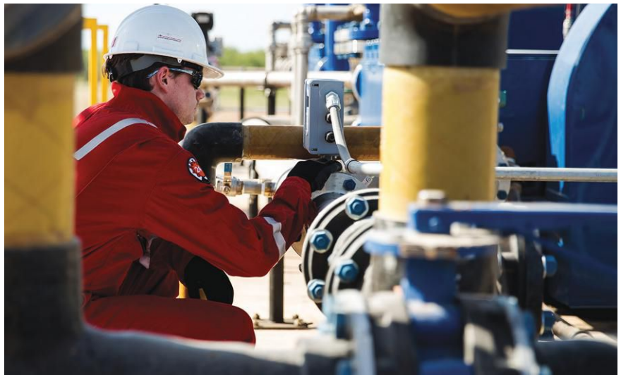
IMAGE 2: Pumping systems with digital and integrated remote capabilities can keep production on schedule. By shedding light on anomalies, adjustments can be made, either remotely or on-site.
