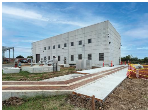
IMAGE 7: The new pump station is expected to last at least 75 years.
