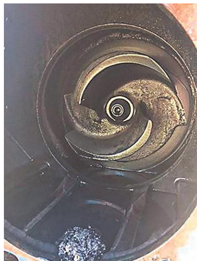
IMAGE 1: Impeller after installation of deragging technology (Image courtesy of Industrial Flow Solutions)
