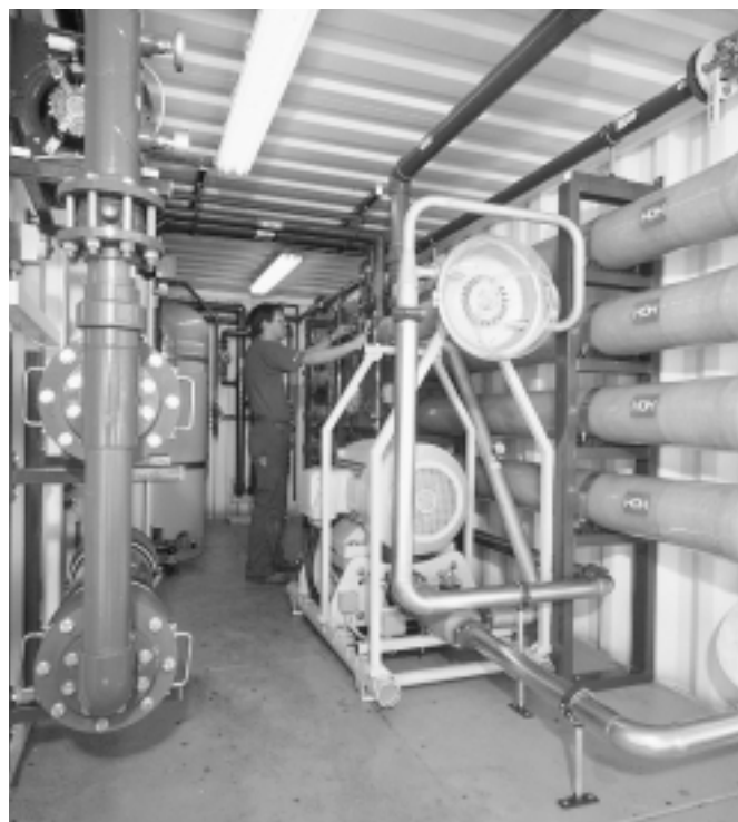
Fig. 58: Reverse osmosis system built into a container with a Grundfos BMET pump
