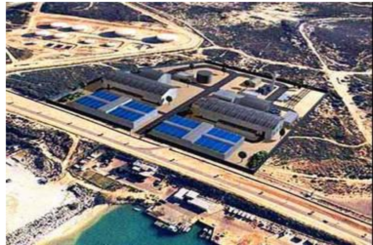
Ashkelon Seawater Reverse Osmosis (SWRO) Plant, Israel Production capacity: 330,000m 3 /day (100 million m 3 /y)
