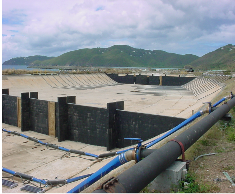
Figure 3.5 Airport Lagoon Treatment Plant during Construction
