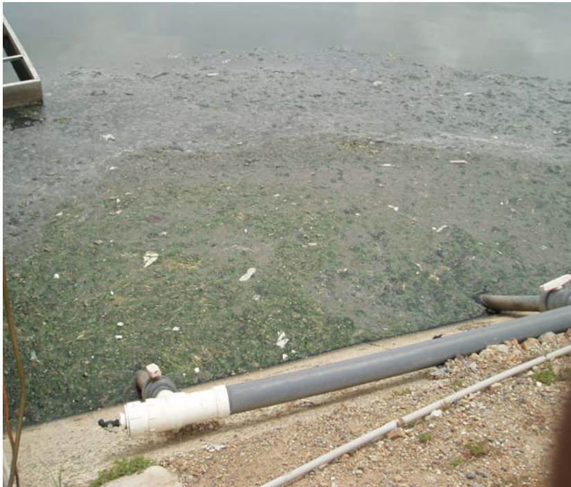
Figure 3.6 Algae Growth in Middle Basin of Airport Lagoon Treatment Plant
