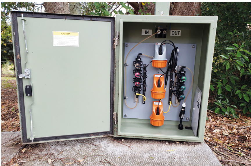
MetriNet, by ATi, is an ultra-low-powered, smart water quality monitoring solution for distribution networks.
