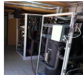
Absorption Chiller (front) & Hydraulic Unit (back)
