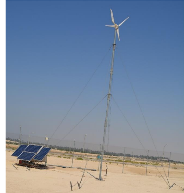
Hybrid (PV-Wind) setup (CER -RI)
