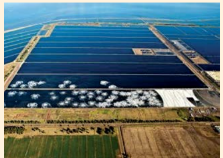
Aerial view of Western Treatment Plant lagoons
