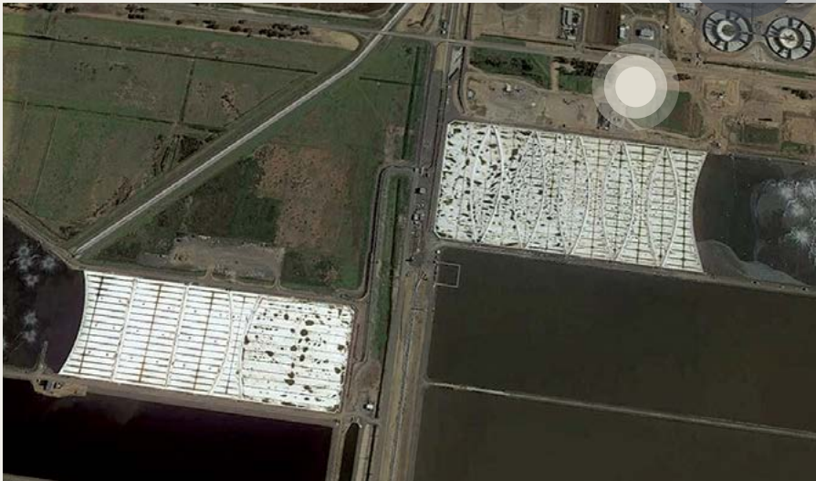
Aerial view of the two covered anaerobic lagoons at the Western Treatment Plant
