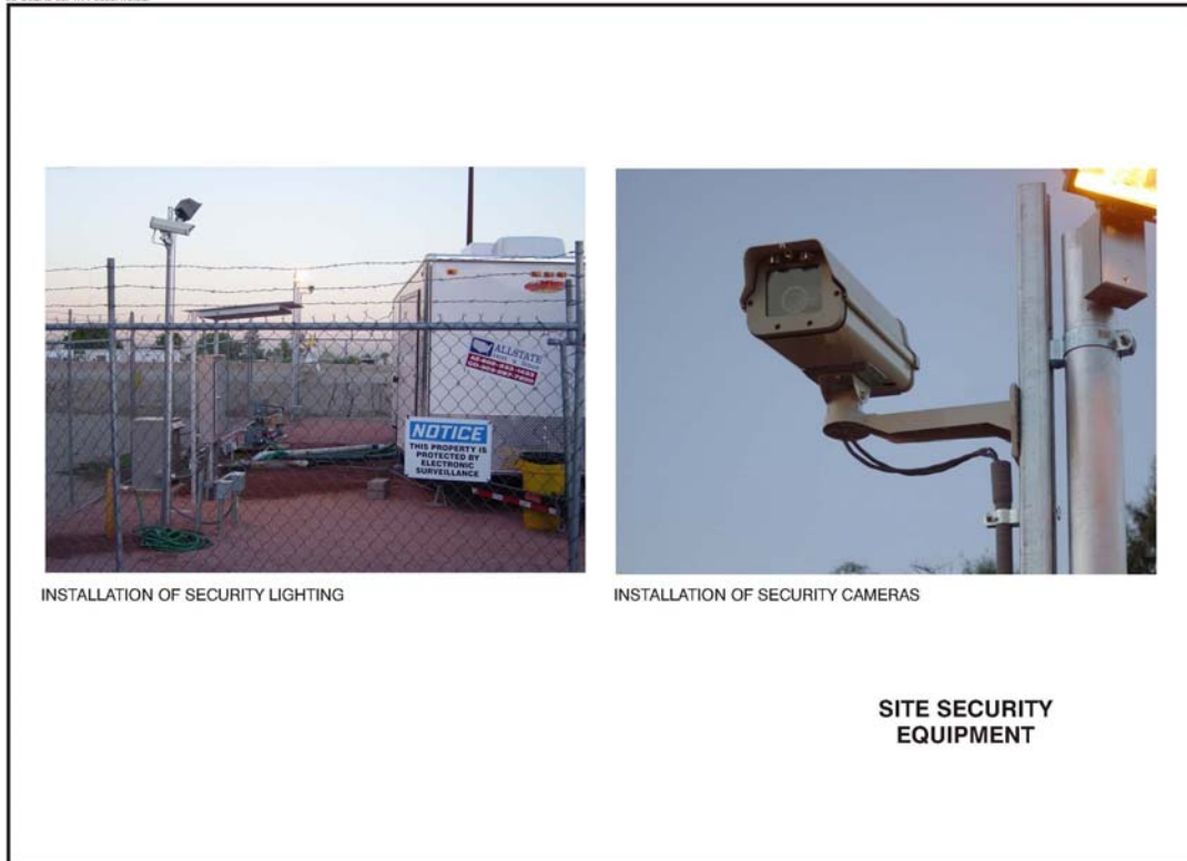
Figure 4.11 Site Security Equipment.
