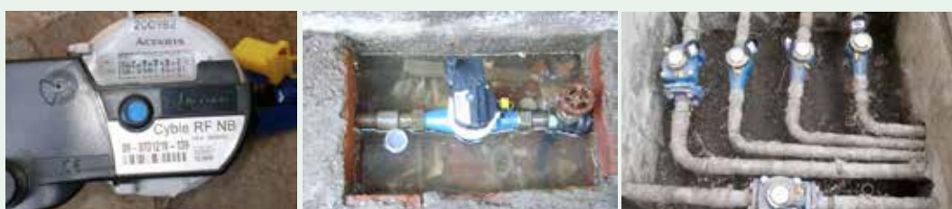
Figure 3. Installed AMR meters in Mumbai (Gomes, 2012)
