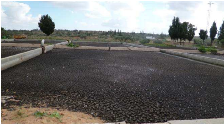
Figure 4: Sewage sludge on drying beds at the WWTP of Ouardanine (with permission of O. Mahjoub 2015)
