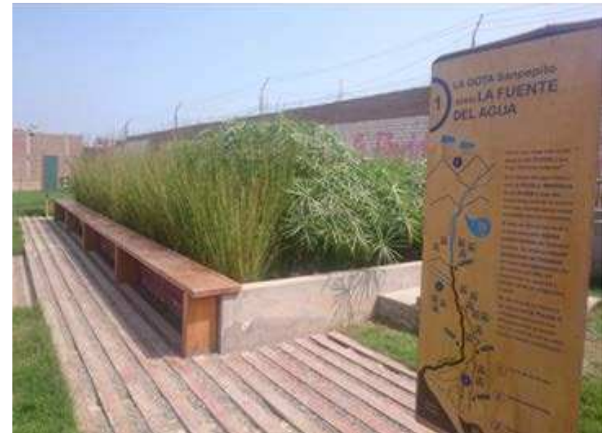
Figure 4: Constructed wetland with the seating bench, wood deck and educational panel about the San José water source, “San Pepito droplet” (Photo: Alexandra Garcia)
