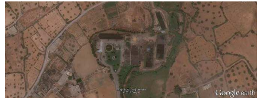
Figure 2: WWTP Ouardanine (Google Earth 2015)
