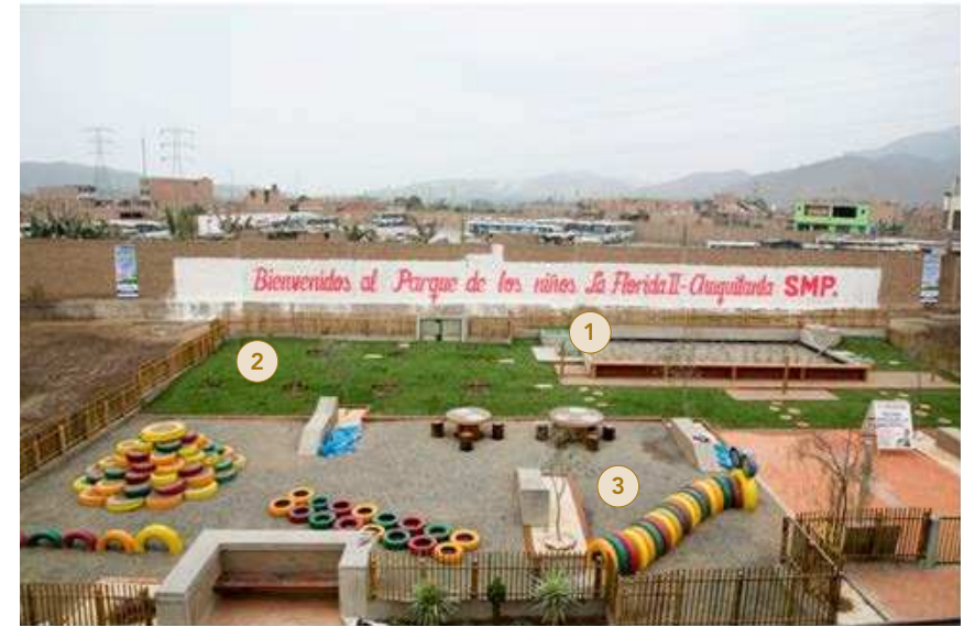
Figure 3: Wastewater Treatment Park – Children's Park on the inauguration day in August 2014, consisting of: 1) treatment system with constructed wetland and reservoir, 2) green recreational area with fruit trees, and 3) play area with dry surfaces (Photo: Evelyn Merino Reyna)
