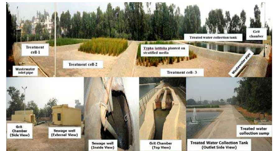
Figure 2: Panoramic view of the proposed (up-scaled) eco-friendly municipal wastewater treatment plant and its components
