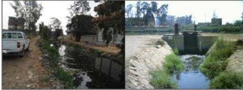
Figure 5: Water at the tail end of two branch canals that receive feeding back from the Nashart and El-Gharibya main drains
