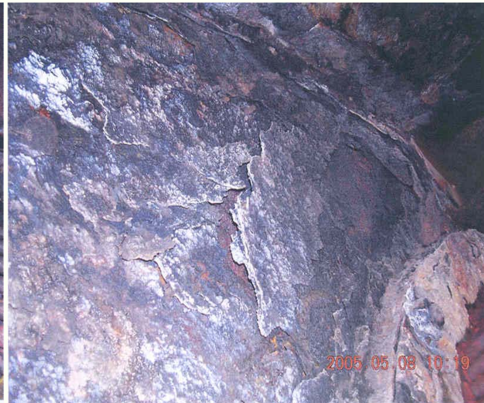
Photo#2 Flash chambers walls
