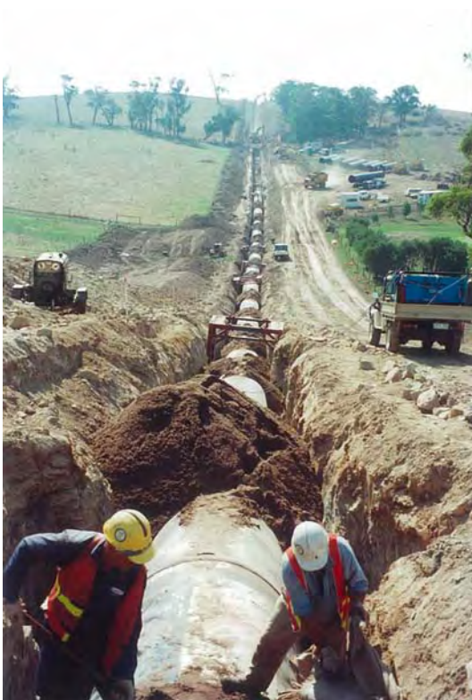
Figure 15 – Construction of a 1700 mm water main in rural and suburban areas
