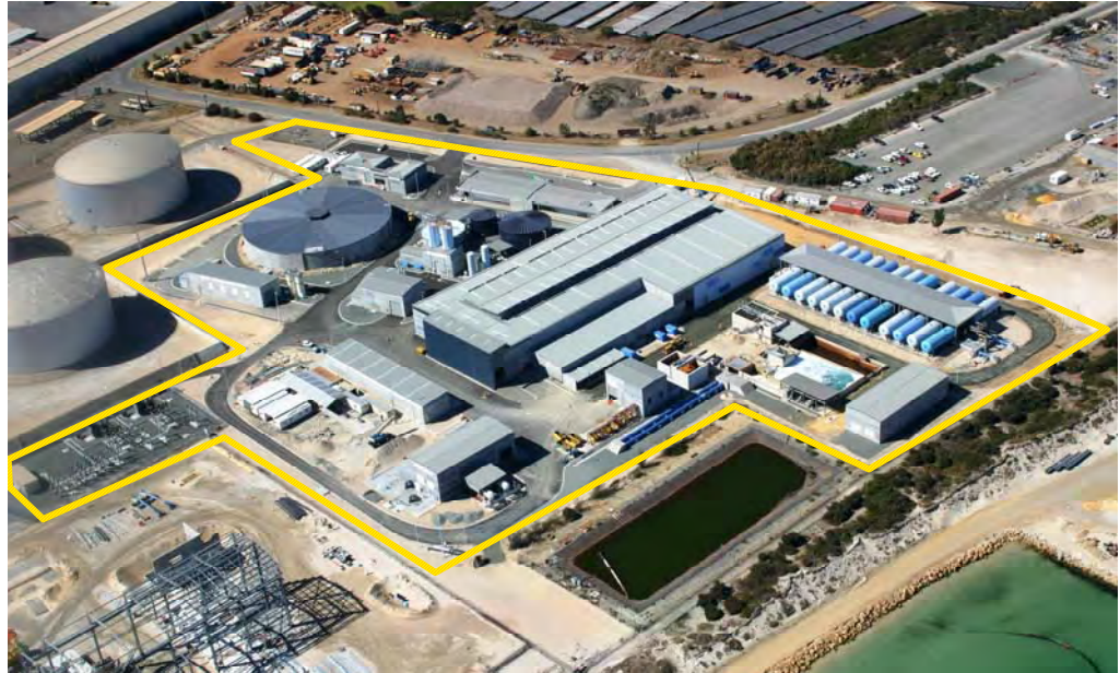
Figure 6 - Perth Desalination Plant 45 GL/year (Permission: WA Water Corp)
