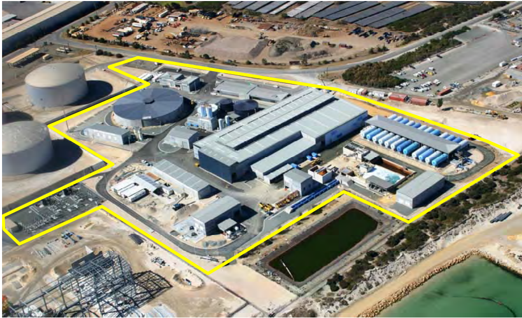
Figure 2 – Perth Desalination Plant 45 GL/y (Permission: WA Water Corp)
