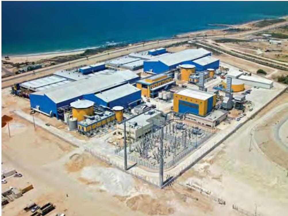
Figure 3 – Ashkelon Desalination Plant, Israel (110 GL/y, co-located with power plant)
