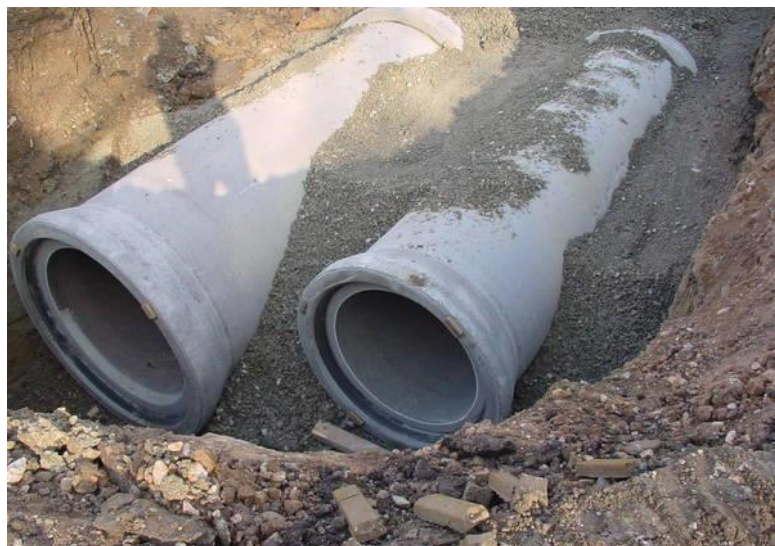
New construction of a separated sewer system in Germany. Source: VILLINGEN-SCHWENNINGEN (2010)
