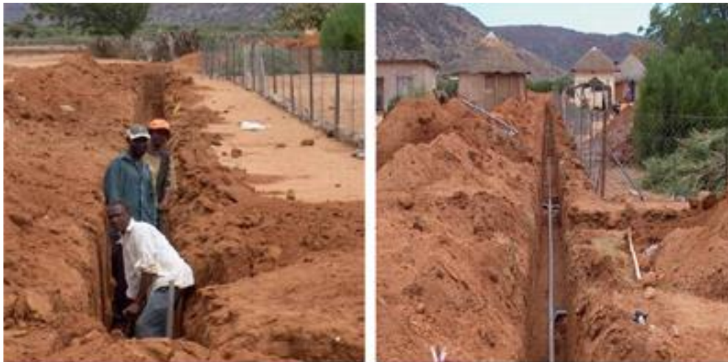
Local workers at construction of a shallow vacuum sewer system.
