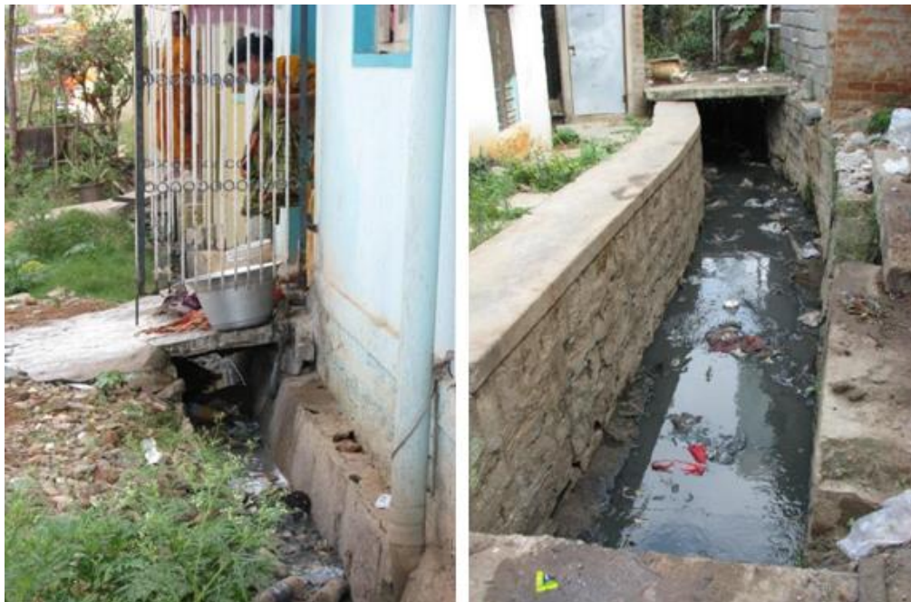
Greywater from laundry (left) and solid garbage which is disposed in open drains (right) pollute water and cause health hazards. Bangalore, Nepal. Source: BARRETO (2009)
