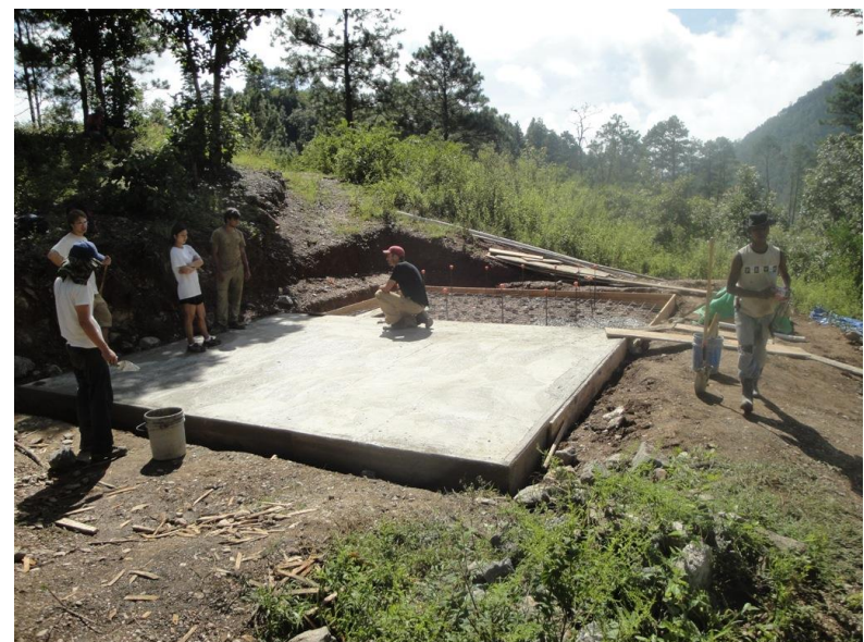
Foundation of a slow sand filter
