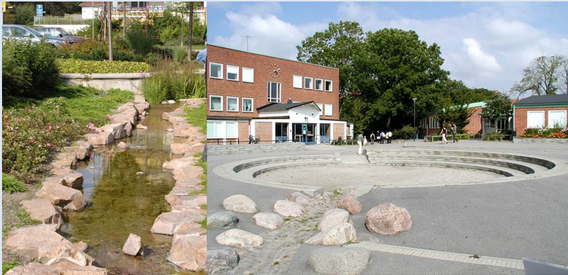
Figure 81. (Left) Stormwater drains are brought to the surface as part of urban landscaping, (Right) A dry retention pond is designed to function as an outside classroom for the adjacent primary school in terms of dry weather, while allowing stored water to infiltrate through its base in wet periods
