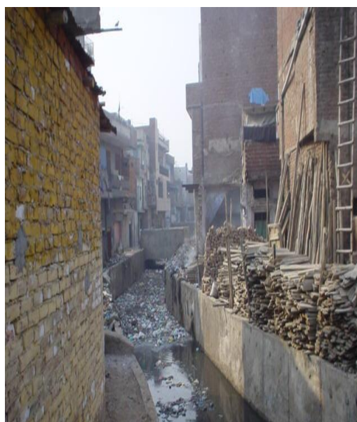
Figure 1.4: Encroachment in storm water drains
