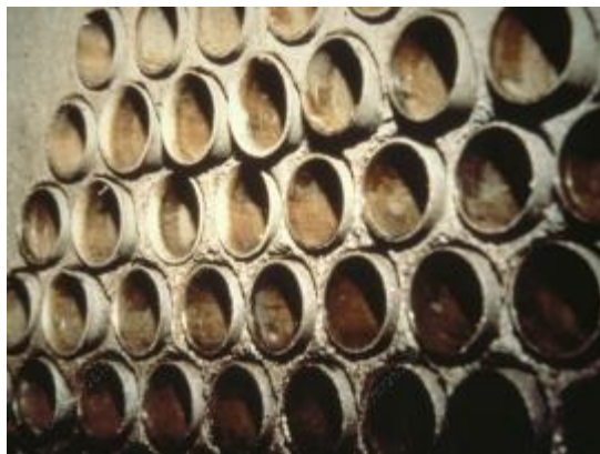
Galvanic Attack – Stainless Tubes with Carbon Steel Tubesheet
