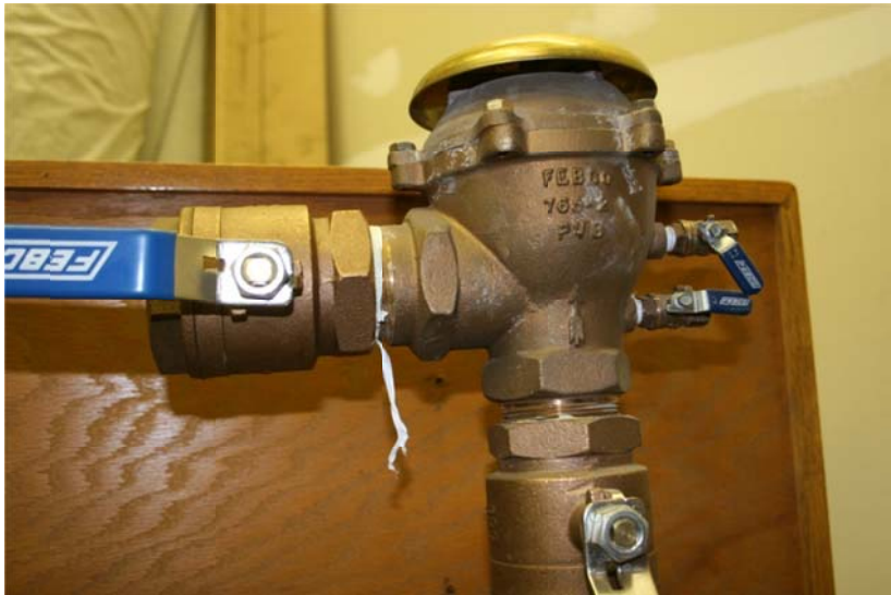
PRESSURE VACUUM BREAKER ASSEMBLY
