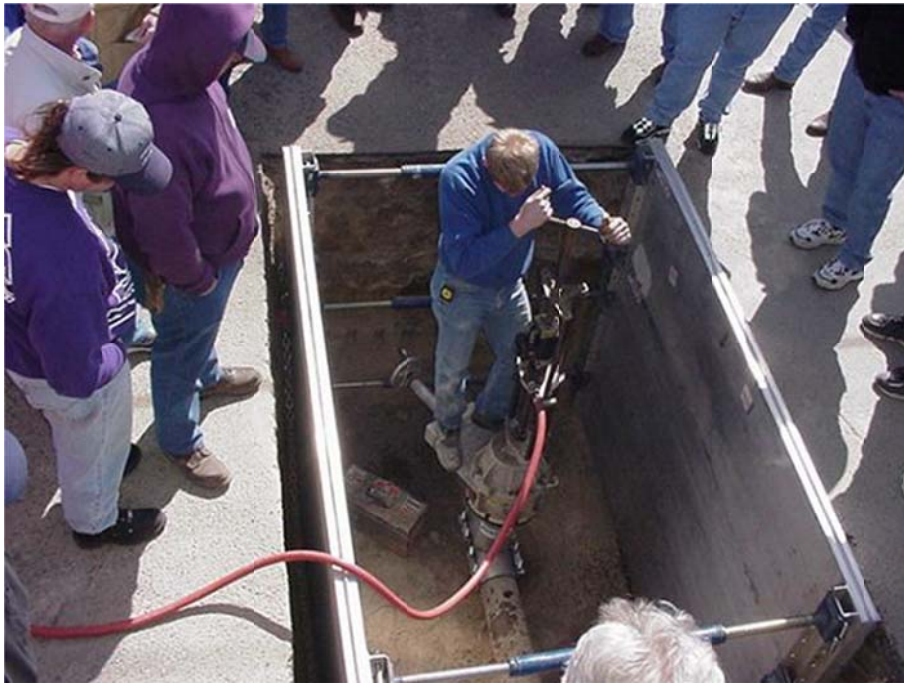
Hydro-Stop valve insertion machine
