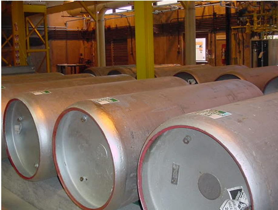
1-ton chlorine containers, rear side of container.
