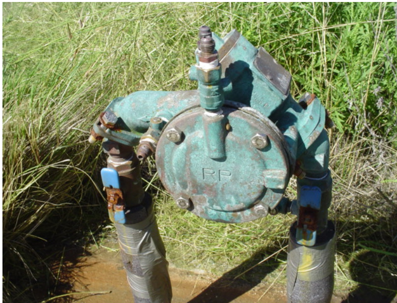
Various Reduced Pressure Principle Backflow Assemblies.
