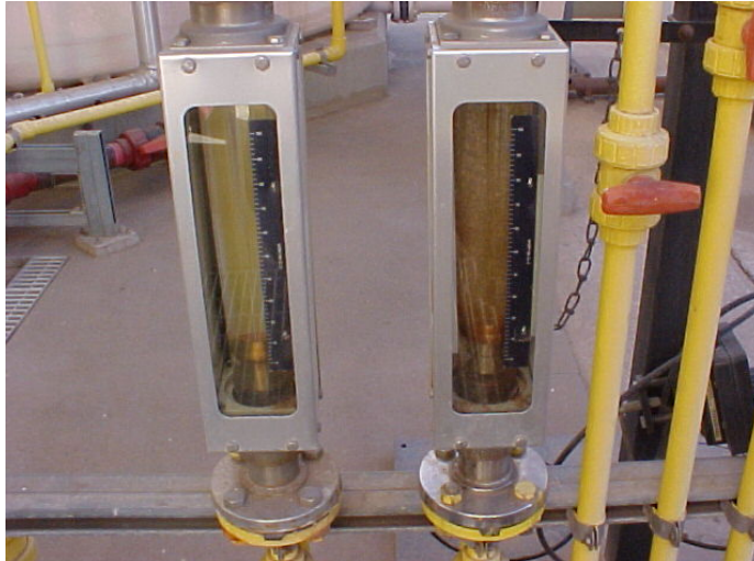
Various Chlorine measurement devices or Rotometers.
