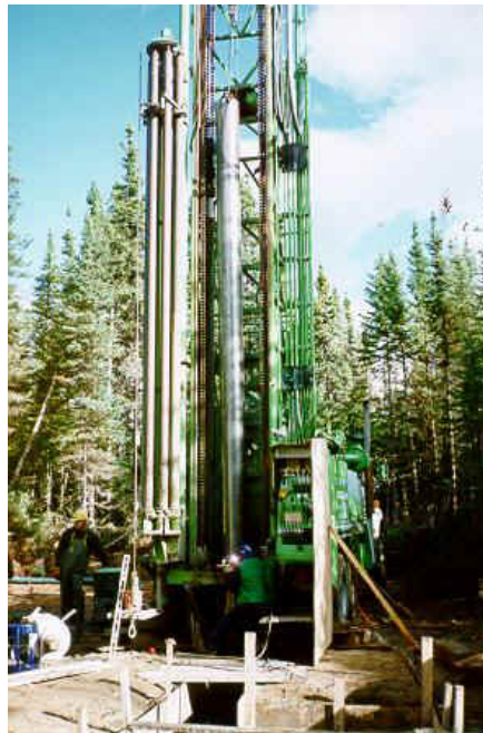
Wire wrapped screen being installed in a well.
