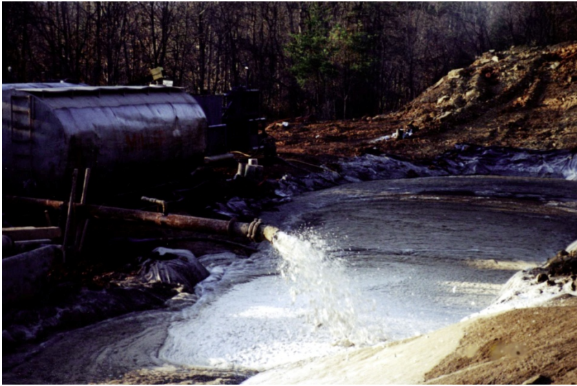
Air Rotary Containment Pit (Notice Foam and Water Truck)
