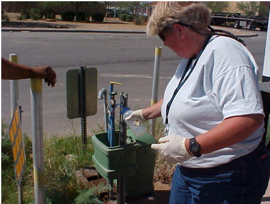
Using alcohol to disinfect a special sample tap before obtaining a sample.
