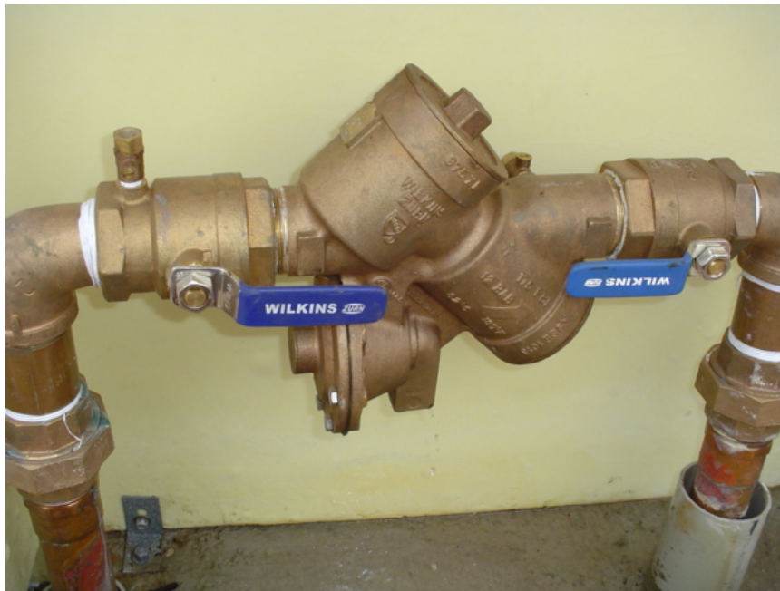
Various Reduced Pressure Principle Backflow Assemblies.
