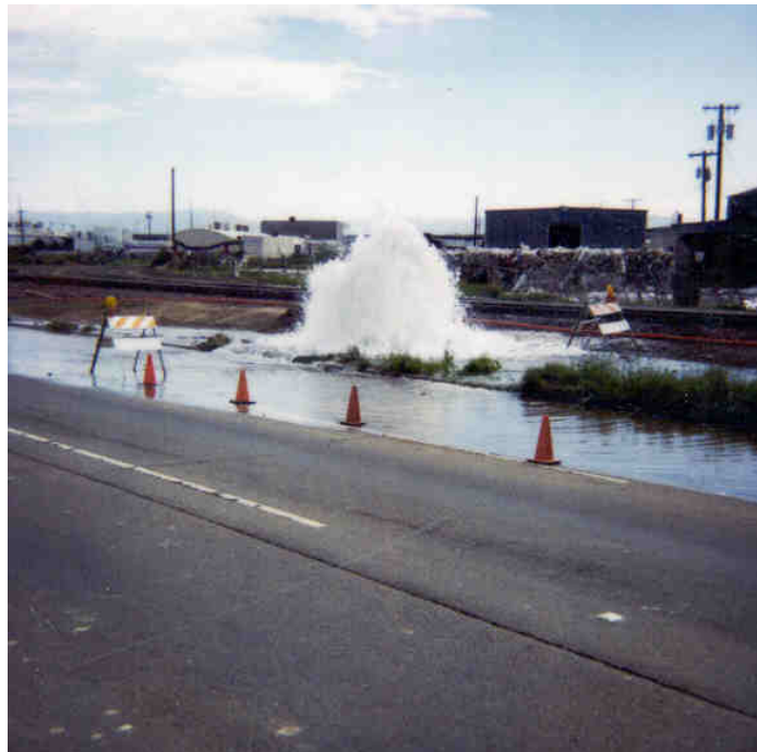
Broken water main, much more larger and stronger leak, more damage, more customers without water. More chance of water contamination.
