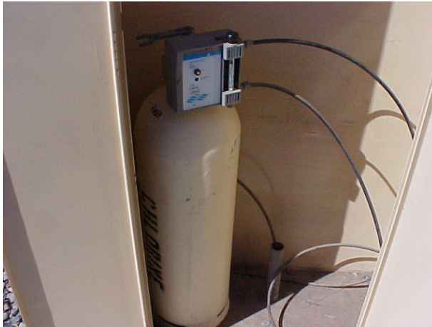
150 pound chlorine gas cylinder. Always tag the empty cylinder and store upright.
