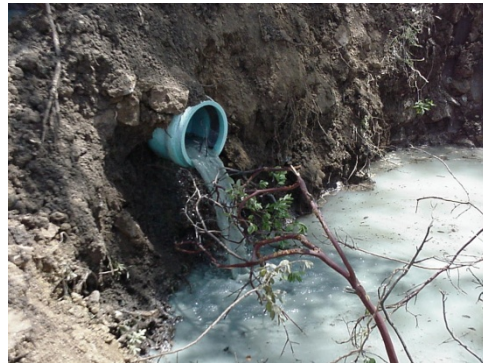
Last Pit (small amount of fines)
