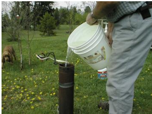
Pouring a Calcium Hypochlorite solution down a well to disinfect the well.
