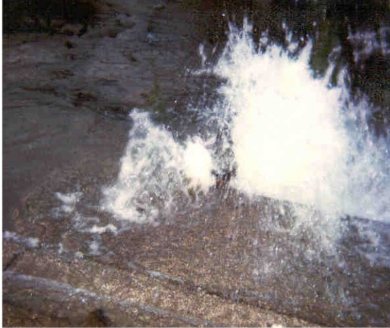
Effects of a broken water service.
