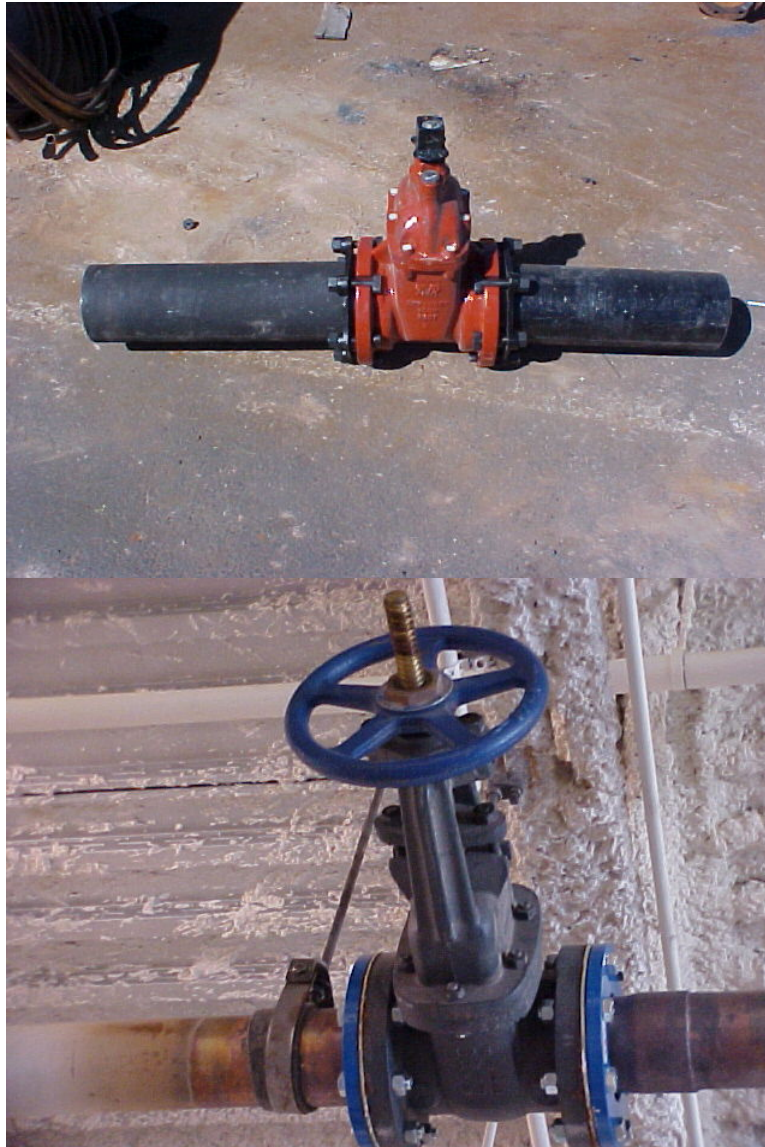
Two different styles of Gate Valves.
