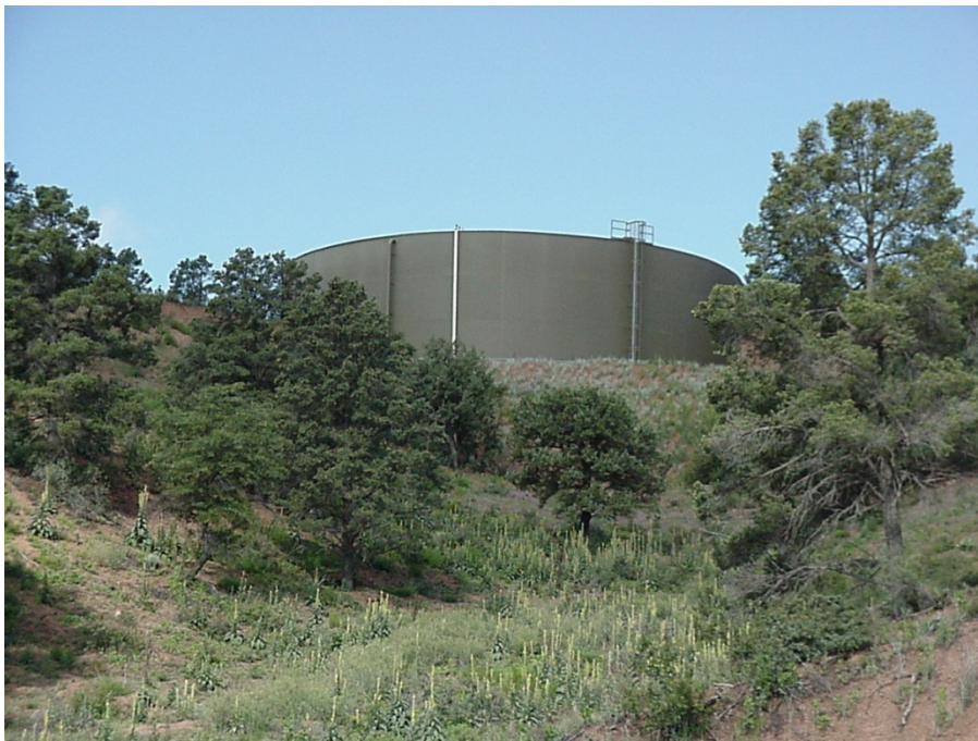
Large steel water storage tank
