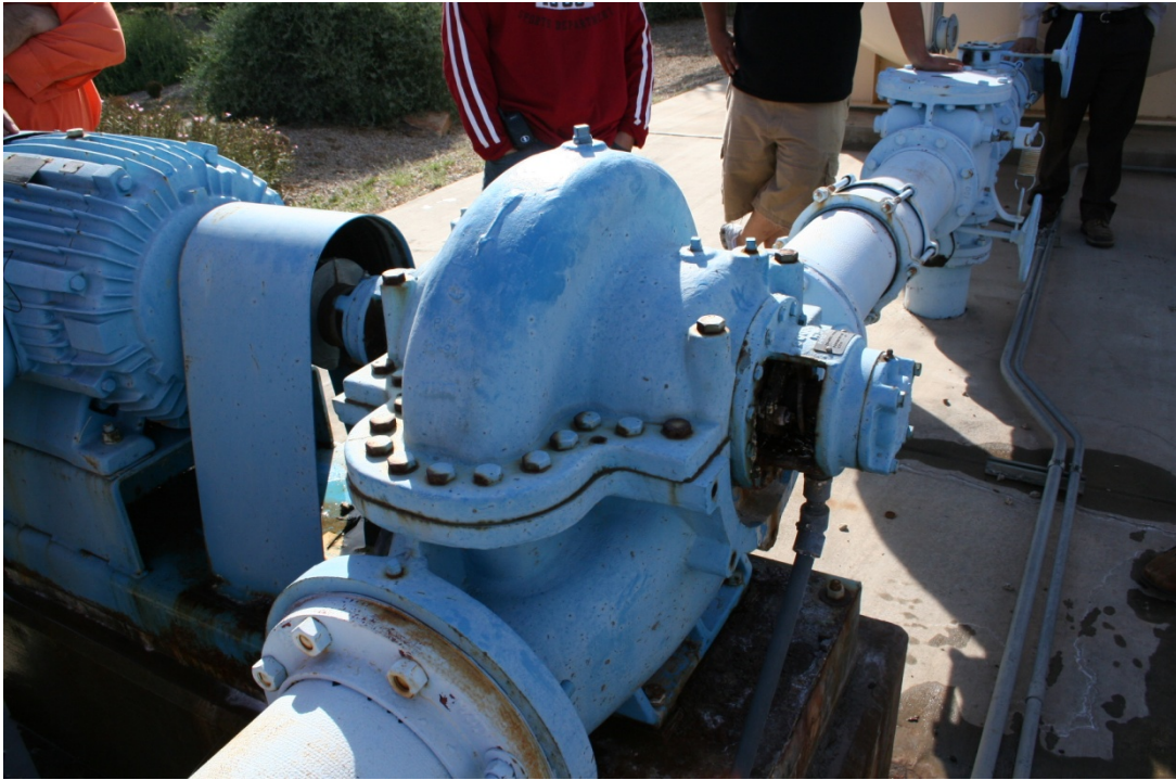
Split-case centrifugal pump.
