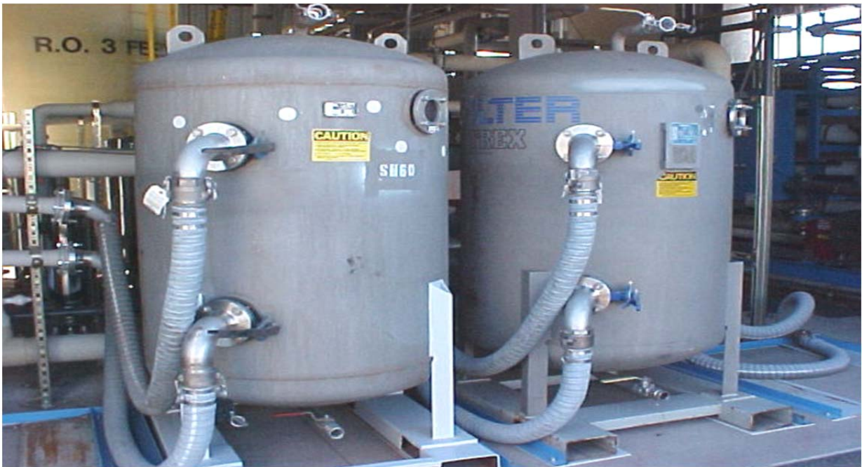
The containers hold the resin for the deionization.
