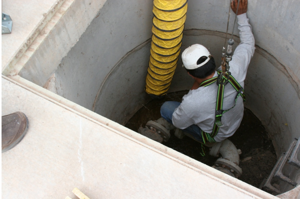
Entering a confined space with proper ventilation.
