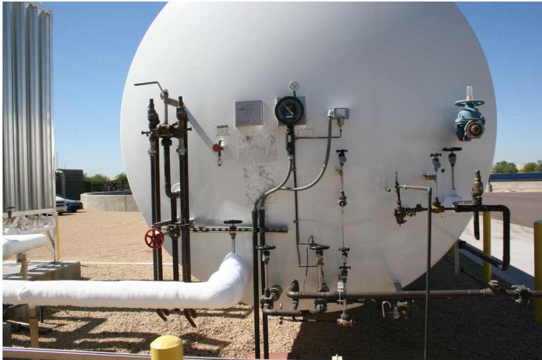
Ozone generator and Oxygen storage tank.
