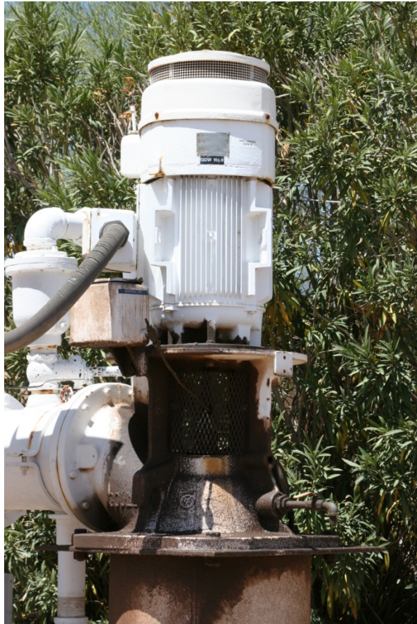
Vertical Turbine well with a mineral oil cooled seal. Mechanical seal bottom.
