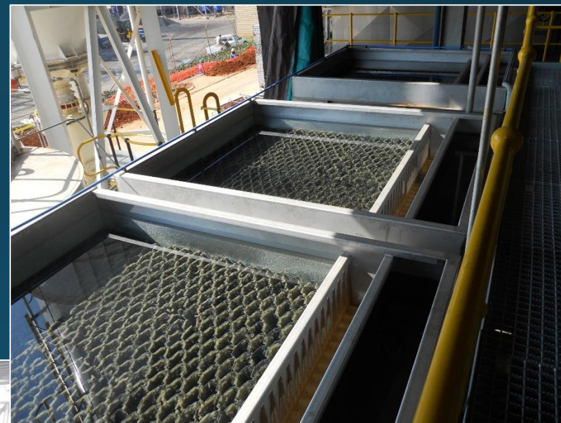
PUR-ALL ZEROZERO Lamella settlers battery
