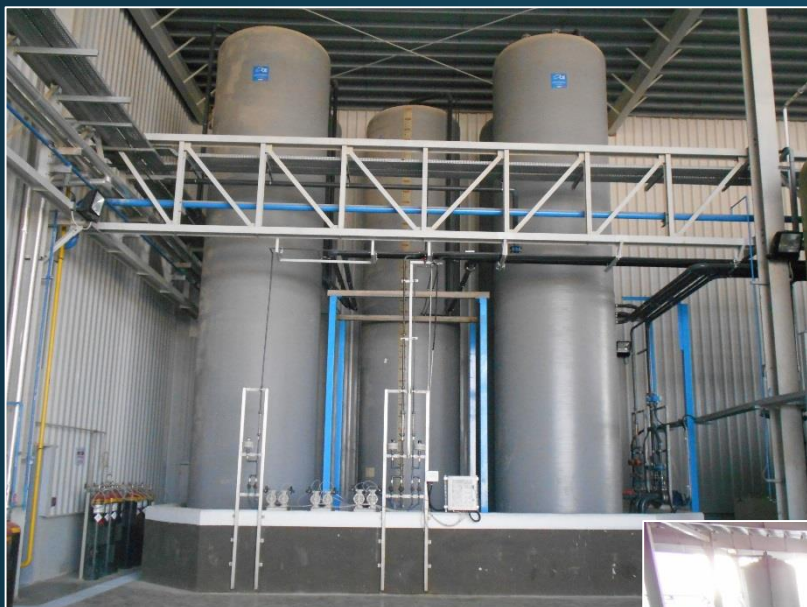
PUR-ALL ZEROZERO Waste water buffer Tanks
