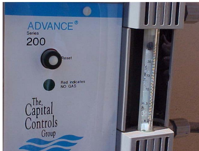
Chlorine measurement devices or Rotameters.
