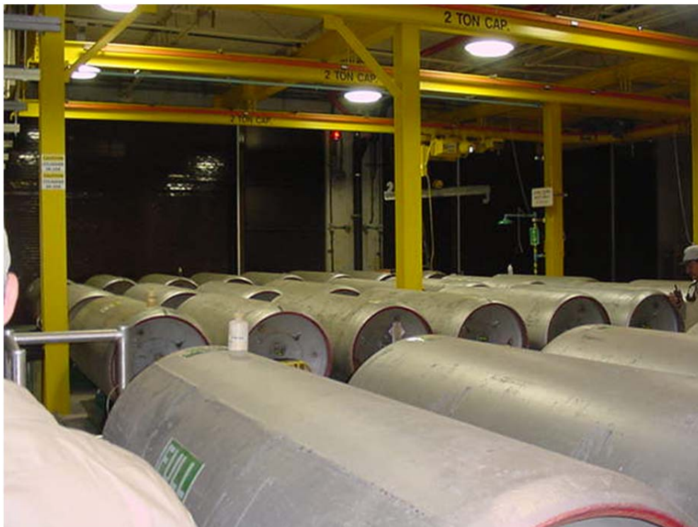
1-ton chlorine gas containers.
