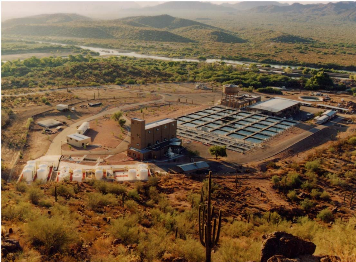
Here is a surface water conventional treatment facility next to a river.
