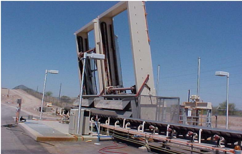
Mechanical bar screen, above photograph. Non-automated bar screen, below.
