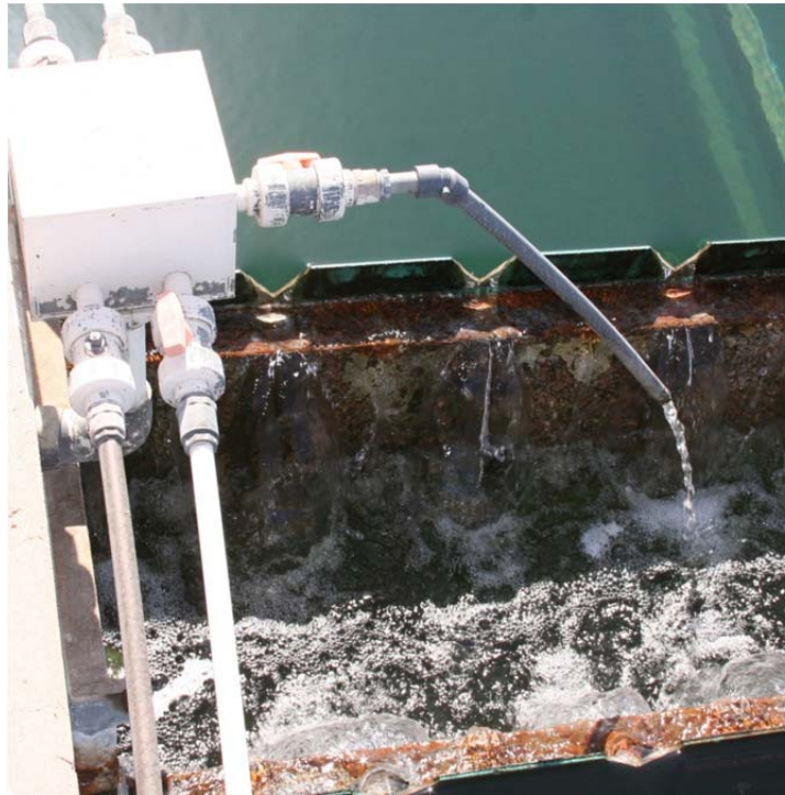
Filter aid being fed at the weirs of sedimentation.
