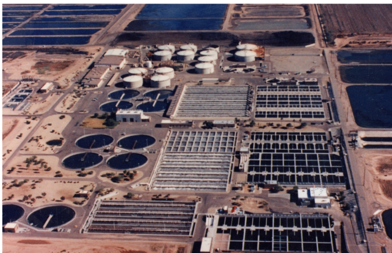
Modern wastewater treatment plant.
