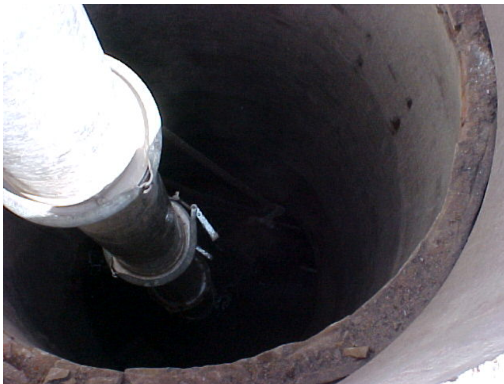
A Vactor clearing a Manhole.
