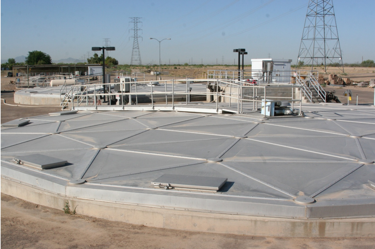
Covered wastewater basins to help prevent or control odors.
