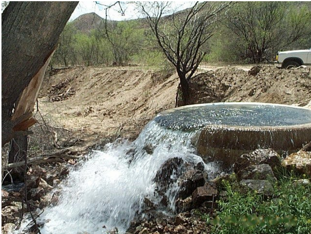
Treated wastewater outfall.
