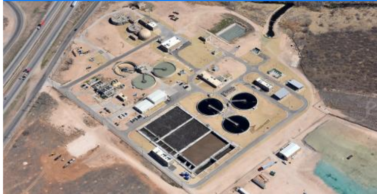
Midland, Texas, Pioneer Water Pollution Control Plant $134M
