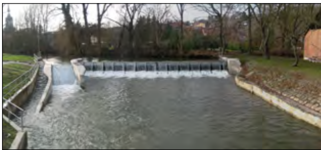
Figure 23: Transverse structure on the Ilm with modern hydropower plant allowing water to flow over and under it, and technical fish pass.
