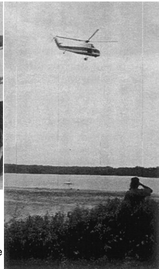
(d) System installation in the lake using a helicopter
