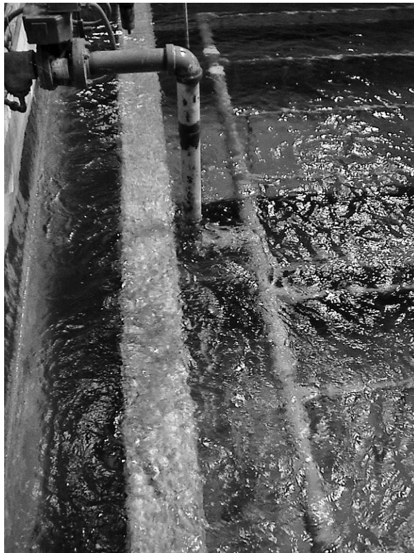
Figure 1-8 Softened, settled, and recarbonated filter influent.
