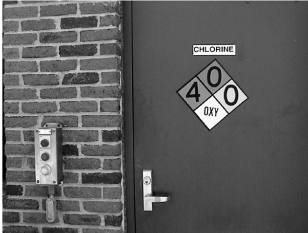
Figure 10-39 Entrance to chlorine feed control room.
