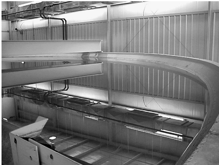
Figure 1-5 Upflow lime slurry contact softener/clarifier.
