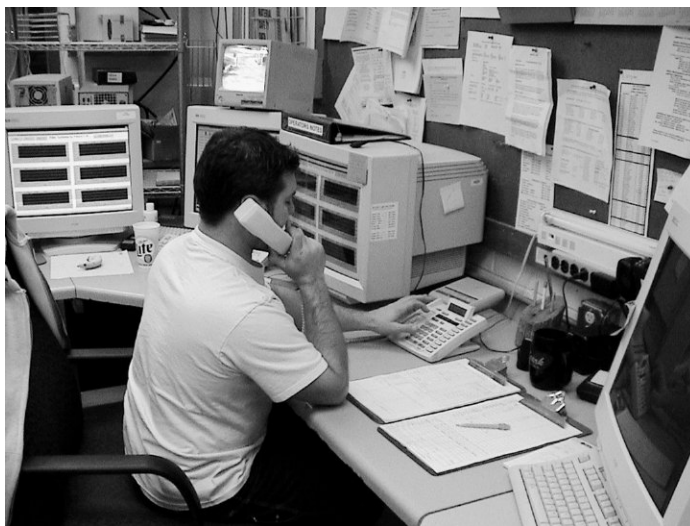
Figure C-1 Operator's Control Room and Monitors.
