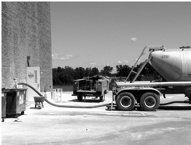
Figure 10-17 Delivery of lime to storage.
