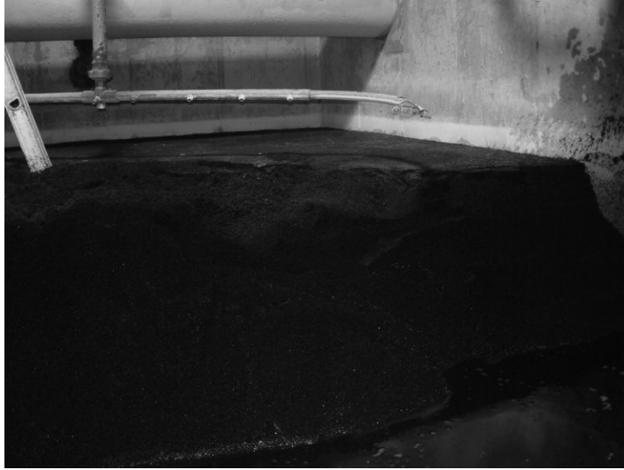
Figure C-46 GAC cap during removal for replacement.
