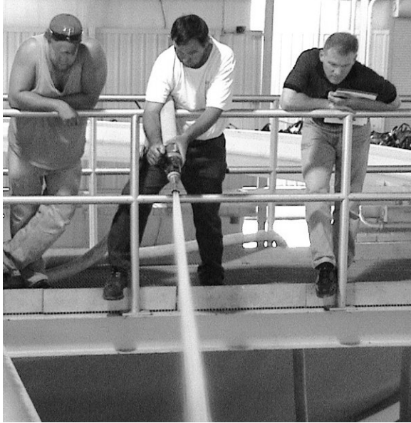
Figure 8-7 Pressure washing.
