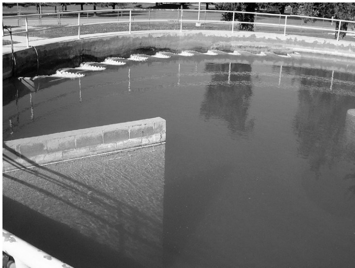
Figure 1-7 Recarbonation basin with serpentine effluent launders.
