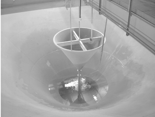
Figure 7-7 Concentrator cone within dewatered ClariCone.
