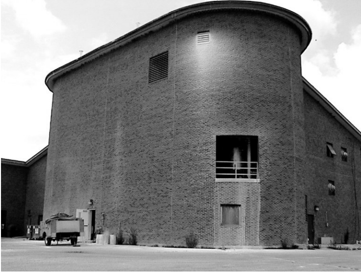
Figure C-23 Lime storage building.
