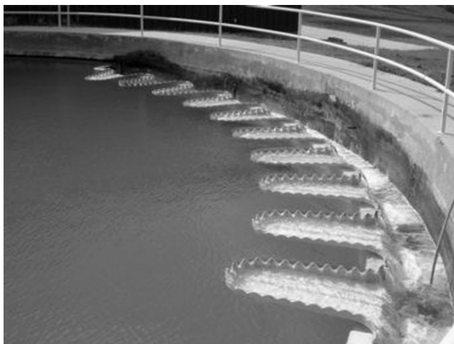
Figure C-40 Serpentine effluent channel.
