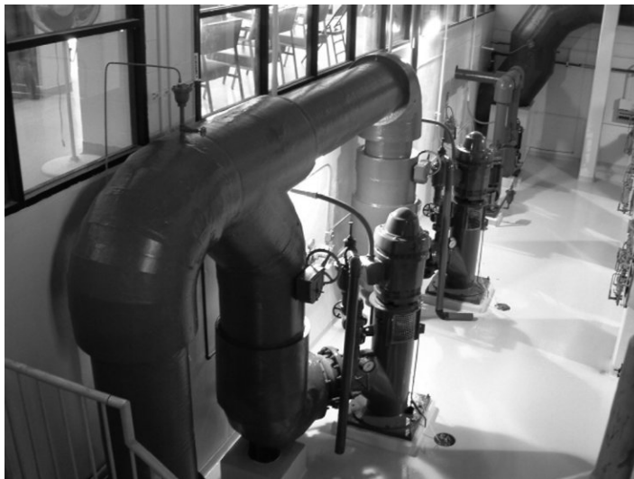
Figure C-5 Plant influent flows are balanced against discharge (production) rates to distribution system and storage.
