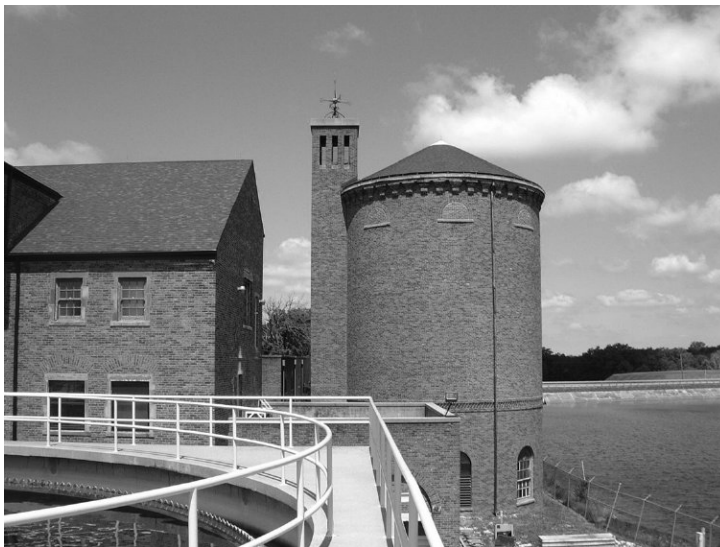
Figure 1-2 Treatment facilities at Lake Bloomington.
