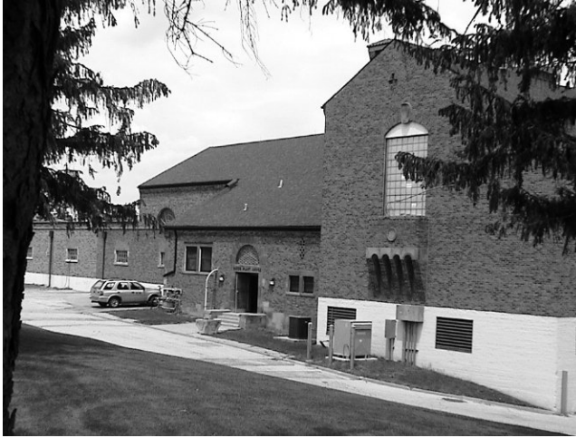
Figure 10-12 1929 Annex (old) Building.
