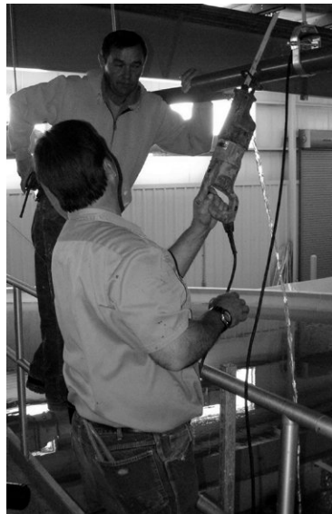
Figure 7-13 Sawing the lime slurry recirculation line.
