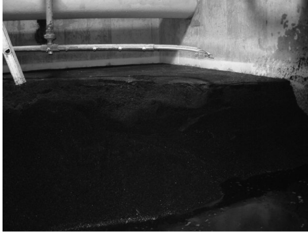
Figure 5-5 GAC cap and surface wash.
