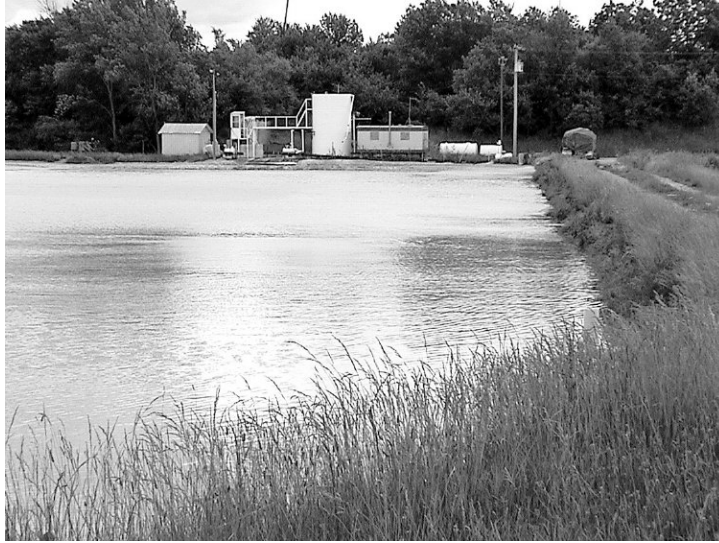
Figure 1-6 Lime softening sludge storage lagoons.
