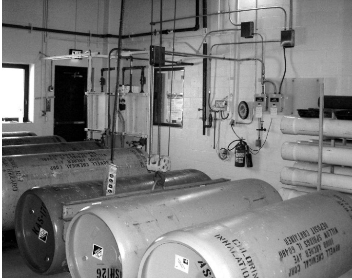
Figure C-12 Special precautions are taken when inspecting chlorine facilities for room ventilation, cylinders in service, rate of cylinder weight loss (feed rate), gas pressure, automatic changeover, alarms, and evidence of leakage (odor).
