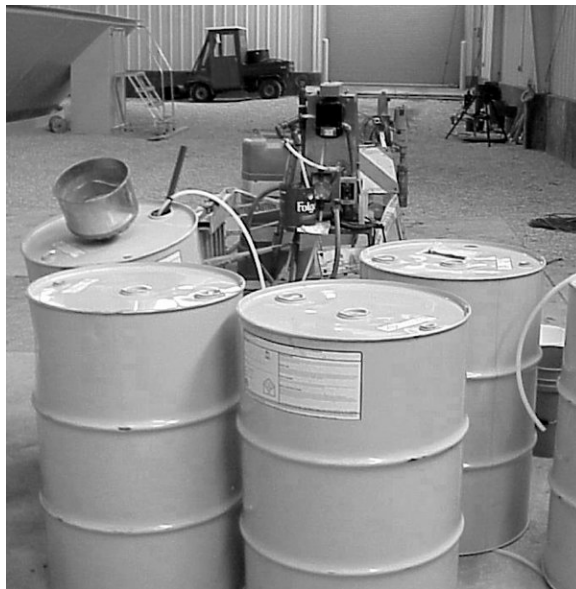
Figure 10-33 Anionic polymer feed to ClariCone influents.
