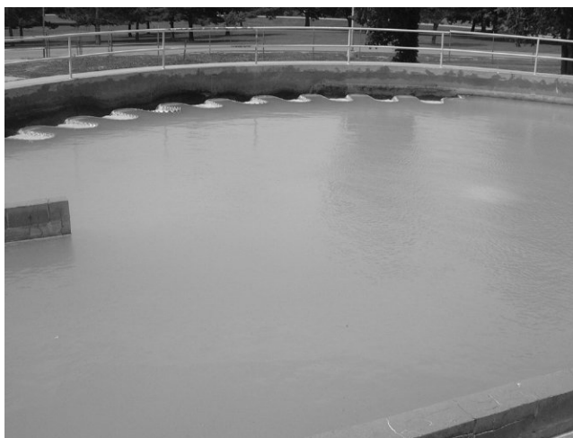
Figure 7-6 Lime overfeed resulting in calcium carbonate post-precipitation.
