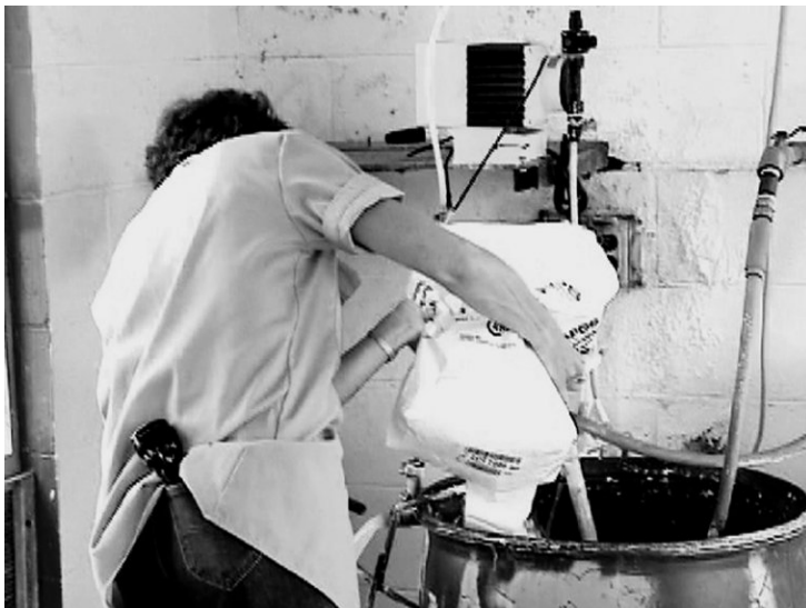
Figure C-15 A 50 lb. bag of polyphosphate “glass” is added to the solution feed barrel daily to prepare a solution of dispersant.
