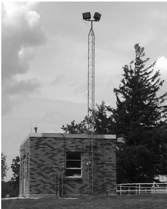
Figure 10-36 Carbon dioxide control building.
