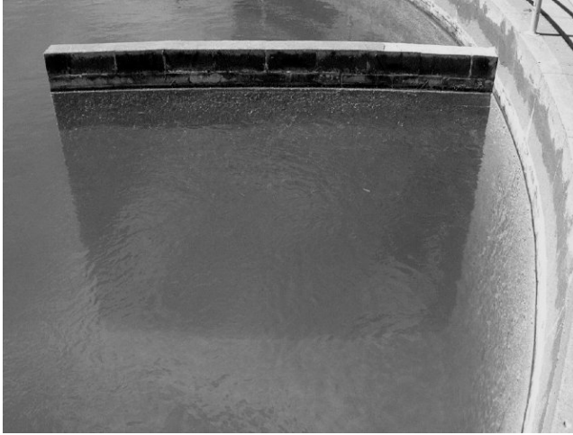
Figure C-41 Recarbonation basin—clear.
