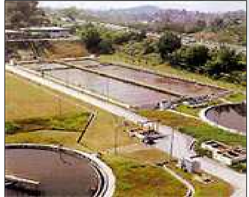
Activated sludge plant
