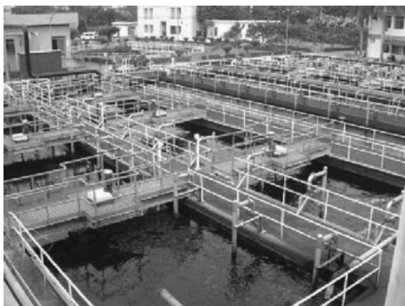
Figure 5.2 Full-scale PACT at Renda Industrial Park (RIP) in TaSheh, Taiwan [3]. (permission received)
