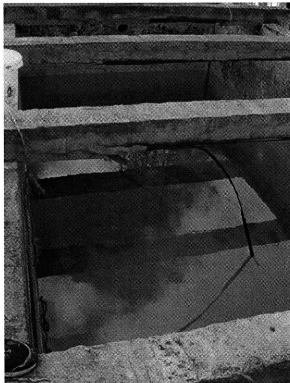
Figure 42 Old cistern tanks at Caneel Bay desalination plant
