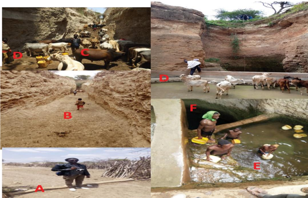
Note: The indicated letters represents Tula structures. A=Gulanta Ela, B=Baqassa Ela, C=Dargula Ela, D=Nanniga (Tula-wells through) E=Faccana (temporary reservoir) F=Qaawa eela (the end source from the tula discharge). (Source: Field visit at Gorile, Dhas and Wachille Tula).
