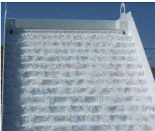
Figure 5-4: Example of cascade aeration unit
