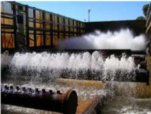
Figure 5-3: Example of spray aeration at Western Australian Groundwater Treatment Plant
