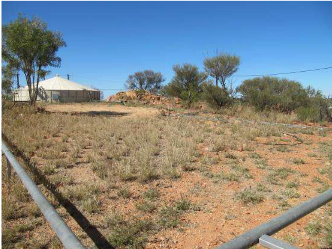
Figure 5–1: Yuelamu Aboriginal Community—raw water tank
