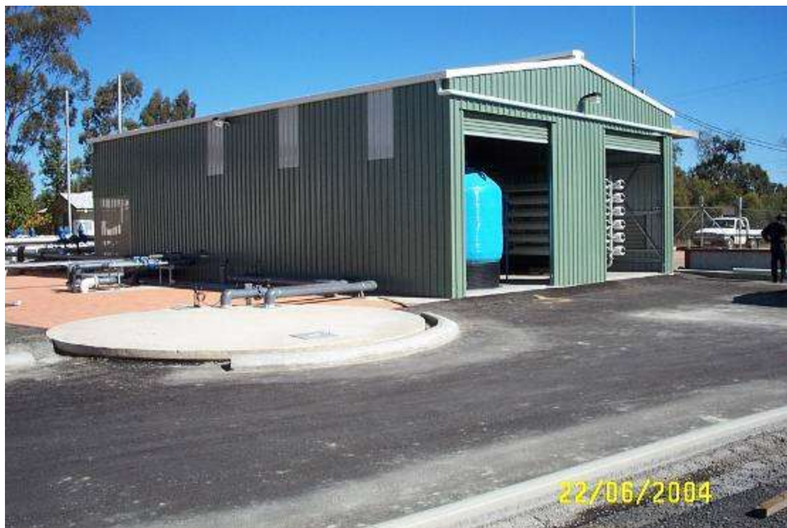
Figure 7–1: Dalby RO water treatment plant #1
