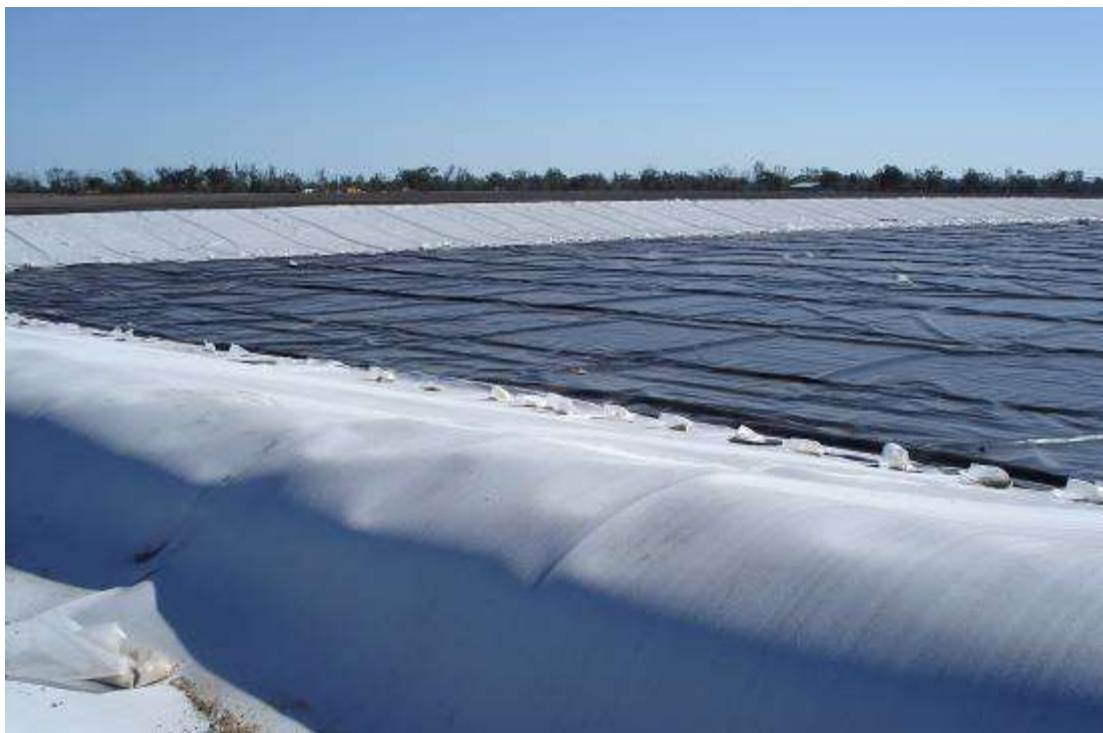
Figure 7–3: Dalby evaporation pond during relining with polyethylene lining
