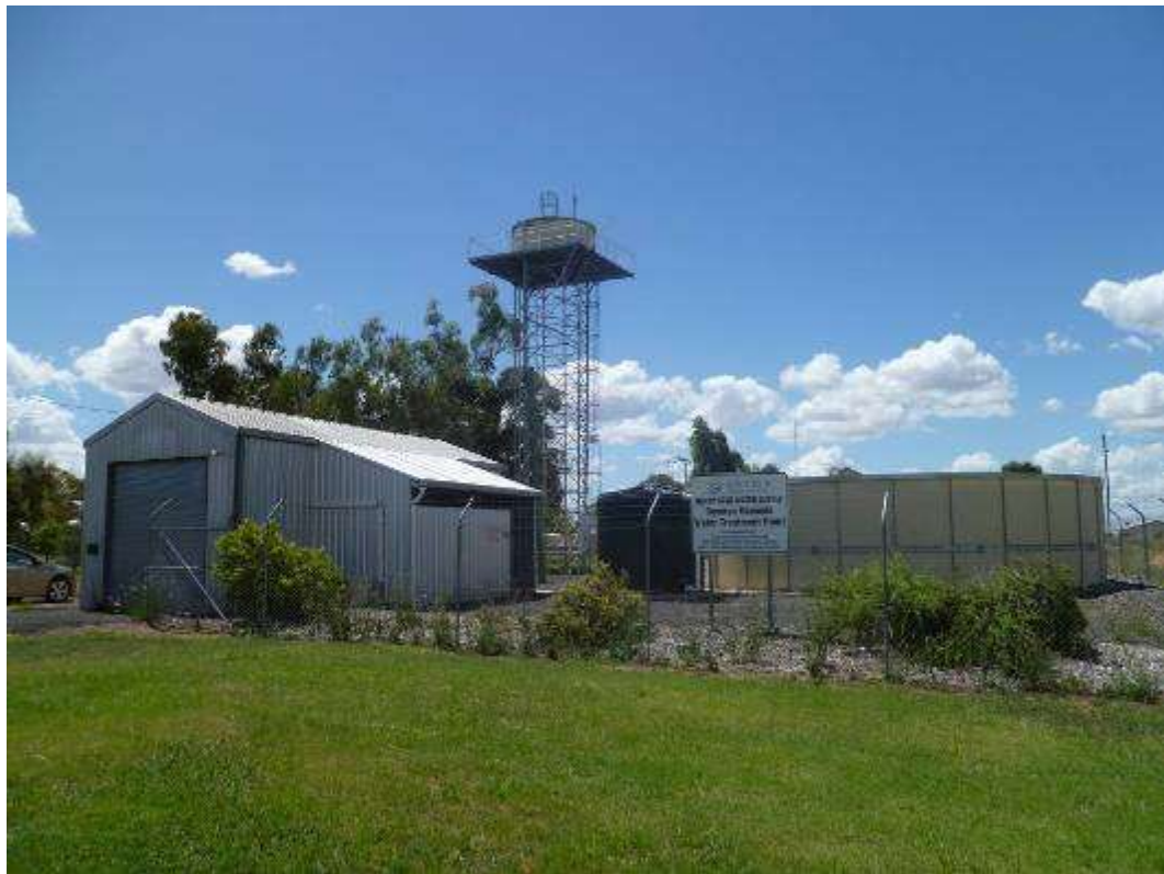
Figure 6–4: a) Typical street in North Star b) North Star water treatment plant
