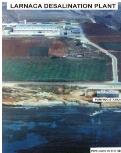
Figure 6: Larnaca Desalination Plant (Taken from Water Development Department )
