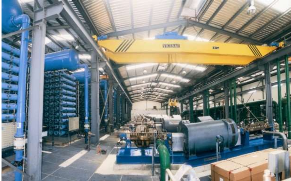
Figure 5: Dhekelia Desalination Plant (Taken from Water Development Department )
