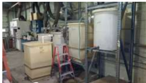
Figure 3 Pilot plant equipment owned by JS Meyer CO
