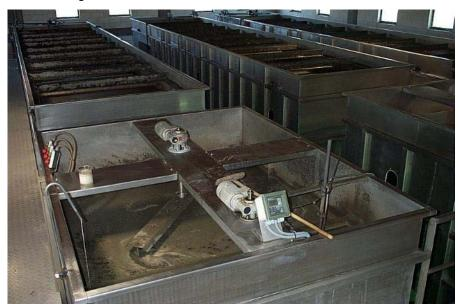
Figure 6.- Physical-chemical process based on coagulation-flocculation + FAD (WWTP Cee - Coruña).
