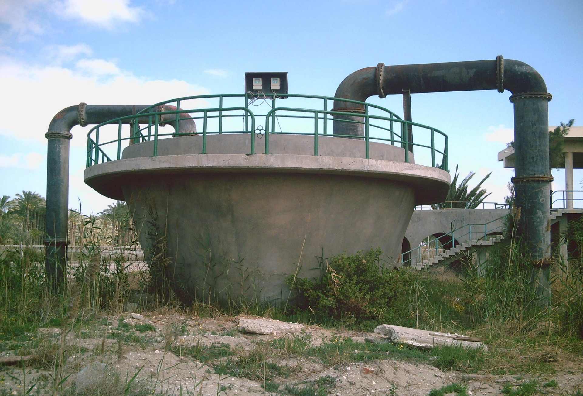
Force mains and deceleration chamber
