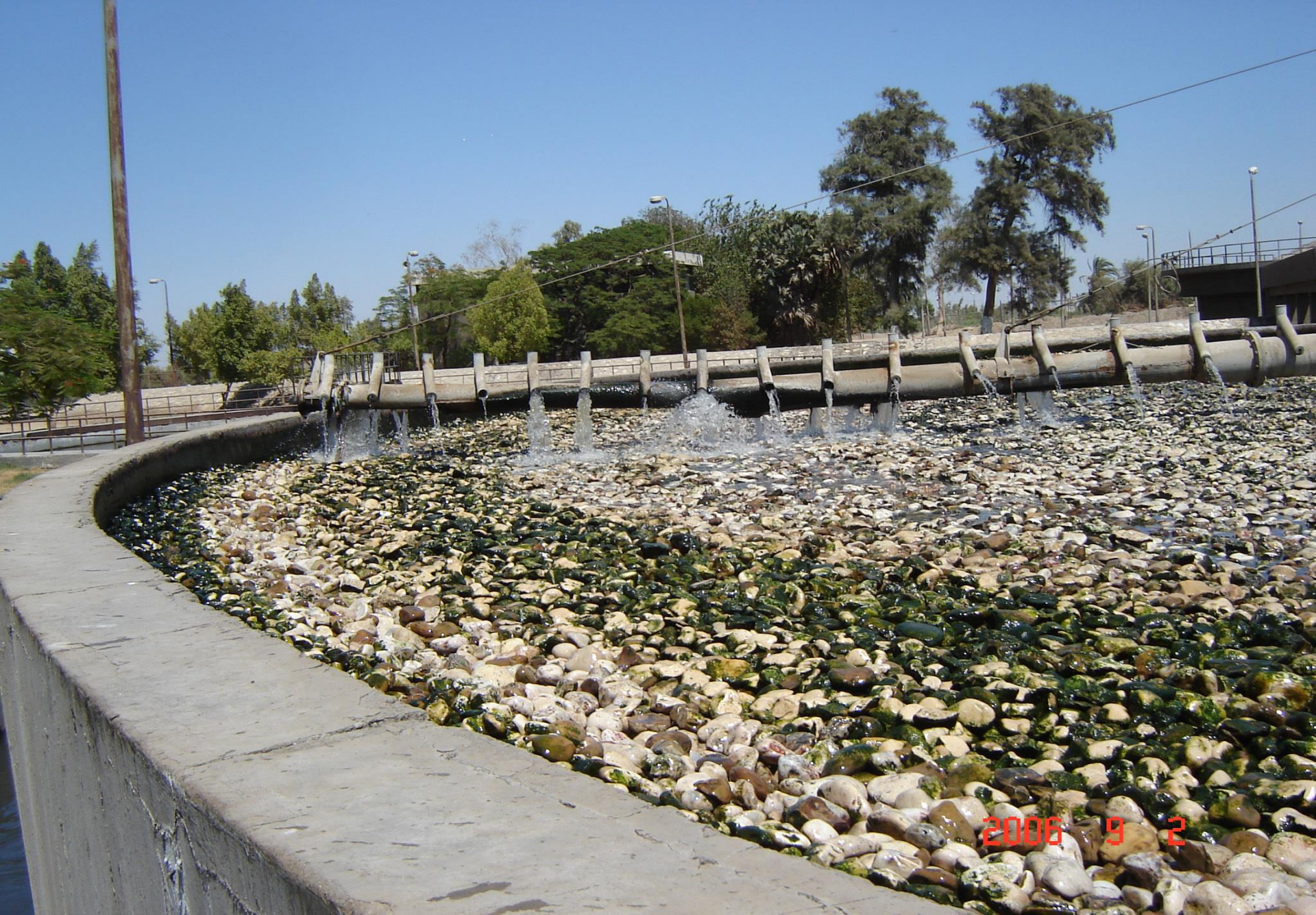
Trickling Filter
