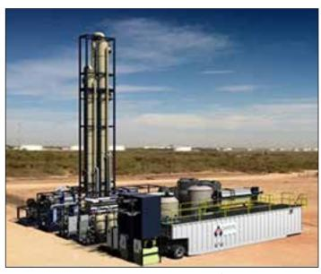
Rendering of company B's forward osmosis process B (adapted from Hancock et al, 2013a and 2013b).
