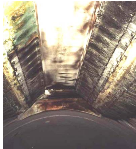
Figure 114. Interior of Double Beam Window in Flue Gas Chamber
