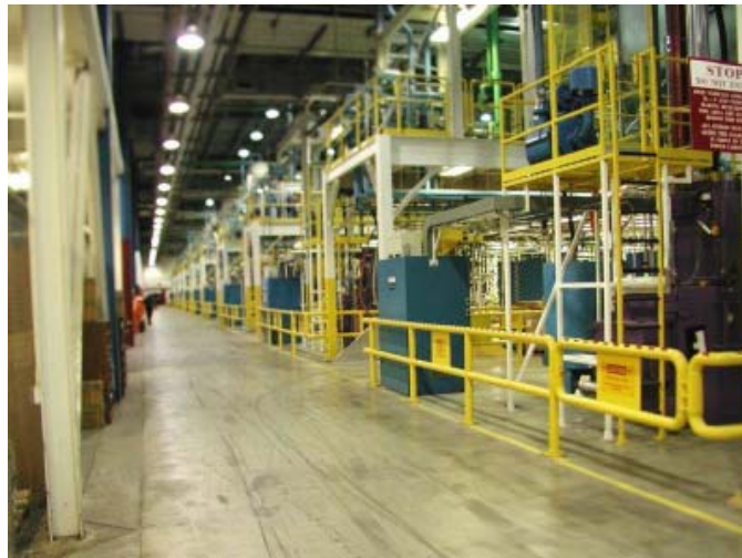
Figure 77. Ten Self-shielded EB Units in One Factory
