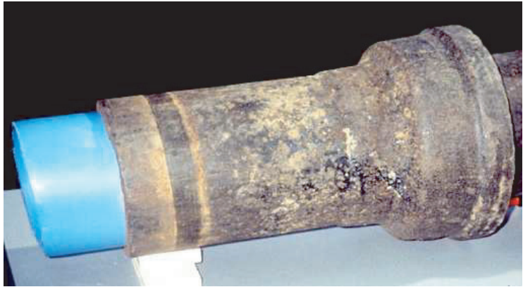
Figure 6.40. Structural relining of an old CI pipe.
