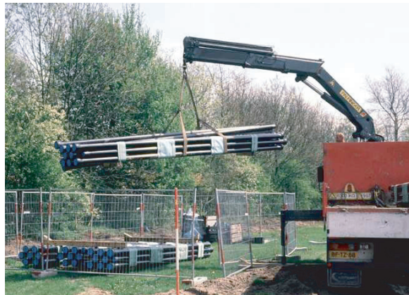
Figure 5.2. Pipe storage on the construction site.
