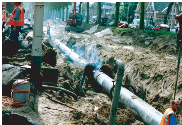
Figure 5.1. Laying of steel pipe.
