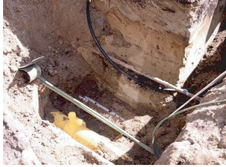
Figure 5.4. Manually excavated trench.
