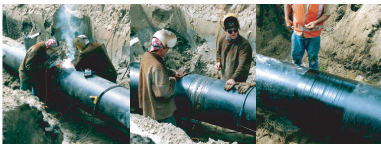
Figure 4.44. Welding of steel pipes.
