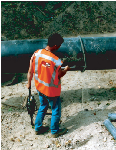
Figure 5.12. Testing of external coating.
