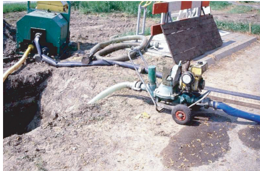
Figure 5.7. Trench dewatering by pumping.
