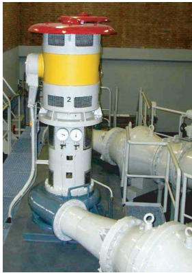
Figure 1.15. Vertical centrifugal pump.
