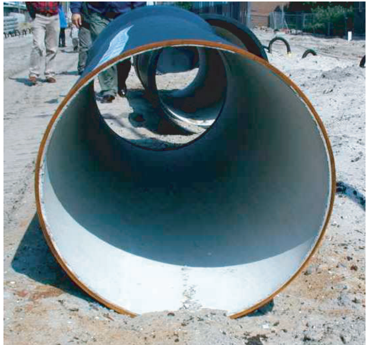
Figure 4.34. Cement lined DI pipe with PE coating.
