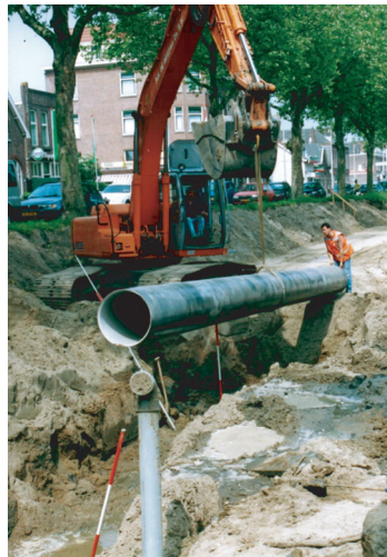
Figure 5.13. Pipe positioning in a trench.
