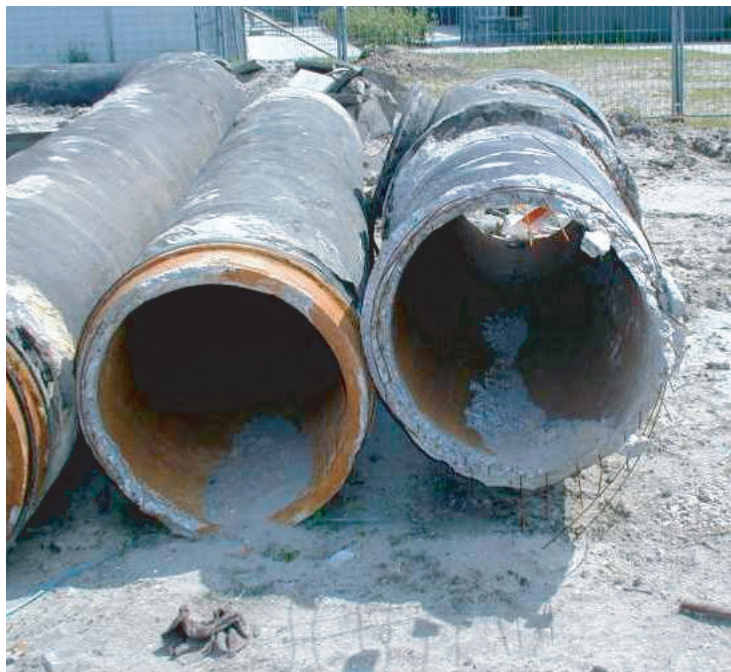
Figure 4.39. Old concrete pipes reinforced with steel net.
