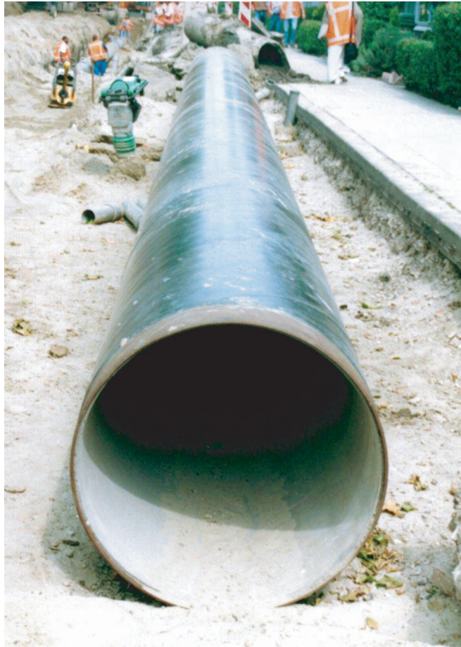
Figure 4.36. Cement lined steel pipe with PE coating.
