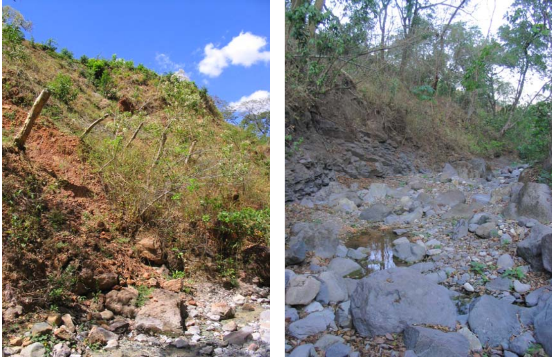
Figure 17. Streamside erosion and low flow conditions near point Sb on the Quebrada El Sabroso.
