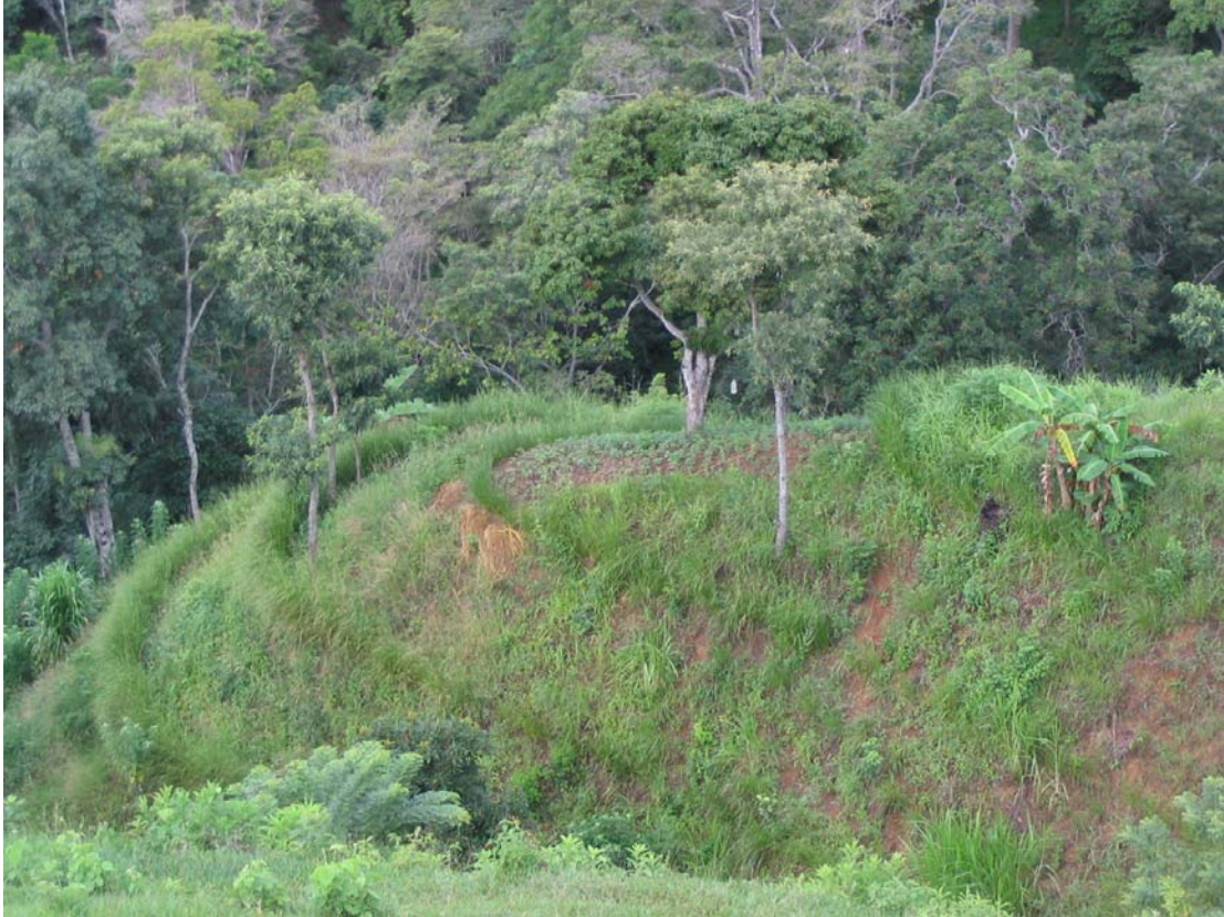
Figure 13. Live grass barriers installed to reduce erosion on steep slopes in the Guanacaure protected area.
