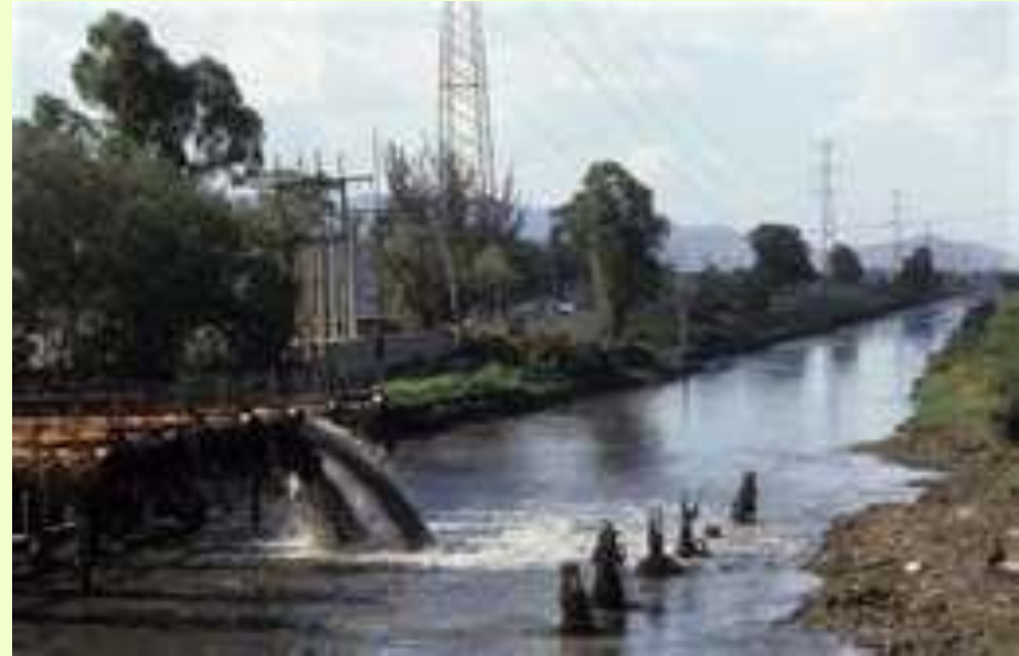
MEXICO. Mexico City. Sewage from Mexico City being pumped into the canal.
