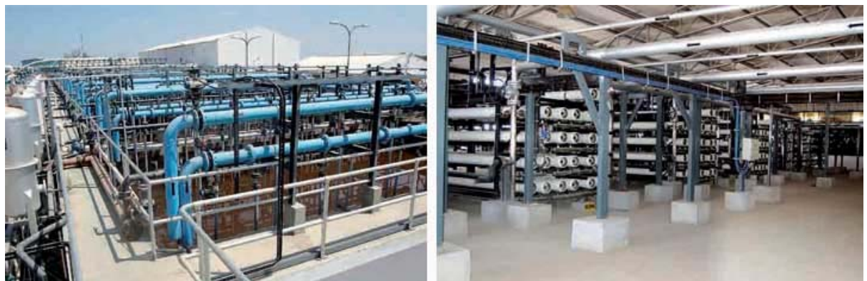
Figure 10. Nanofiltration and reverse osmosis systems in a Zero Liquid Discharge CETP in Angeripalayam, with high contribution of textile effluents, in Tirupur (India).
