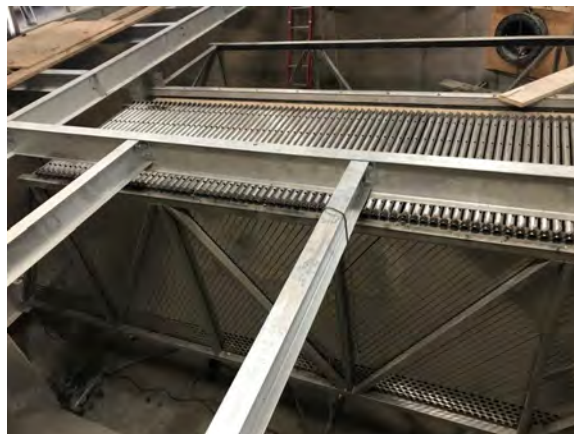
Figure 5 – Plate Settlers
