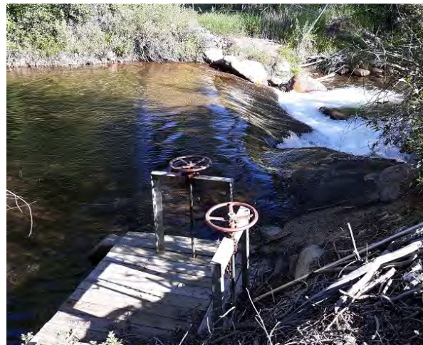
Figure 2 – Existing Intake Structure
