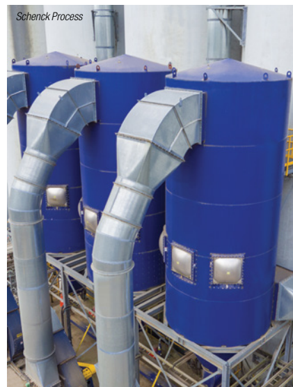
FIGURE 5. MCF PowerSaver technology uses a positive-displacement blower package, which requires 50% of the energy of a typical pulse-jet system, providing a significant energy savings
