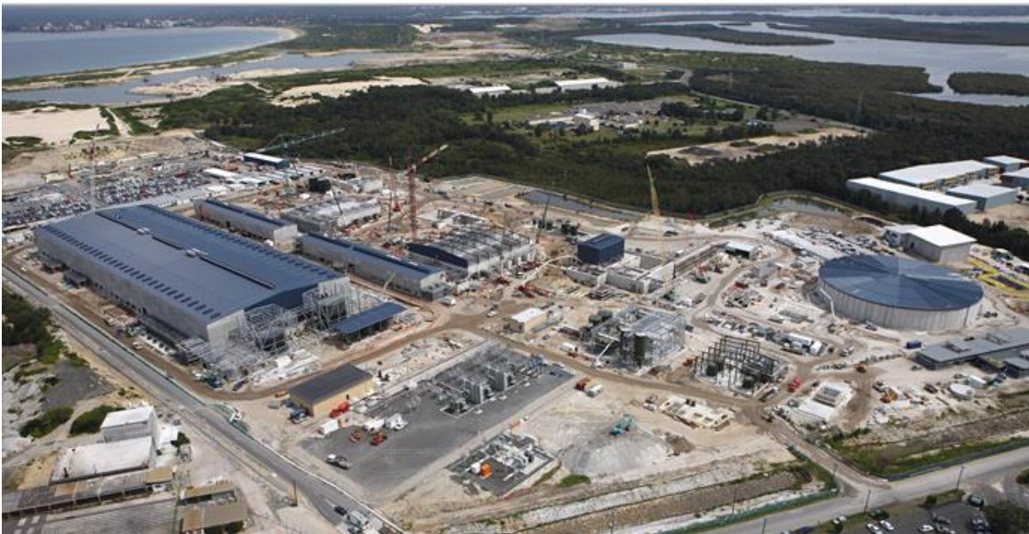
Figure 33: Sydney Wind-RO plant during construction [51]
